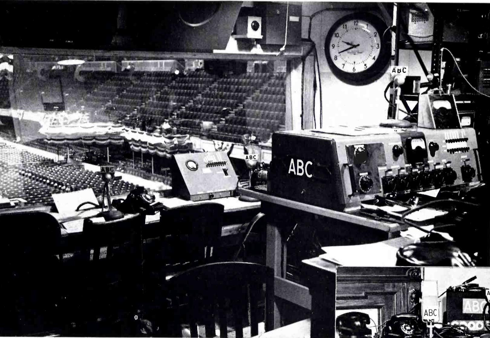
ABC's CONVENTION HALL AM/FM CONTROL BOOTH is pictured here. Equipment position, at right, sported a modified RCA 76-B2 Console. RCA 88-A Microphones were used at the announce positions along the table in front of the window. Small picture at the right shows a corner of the ABC sound studio at the Bellevue-Stratford Hotel.
