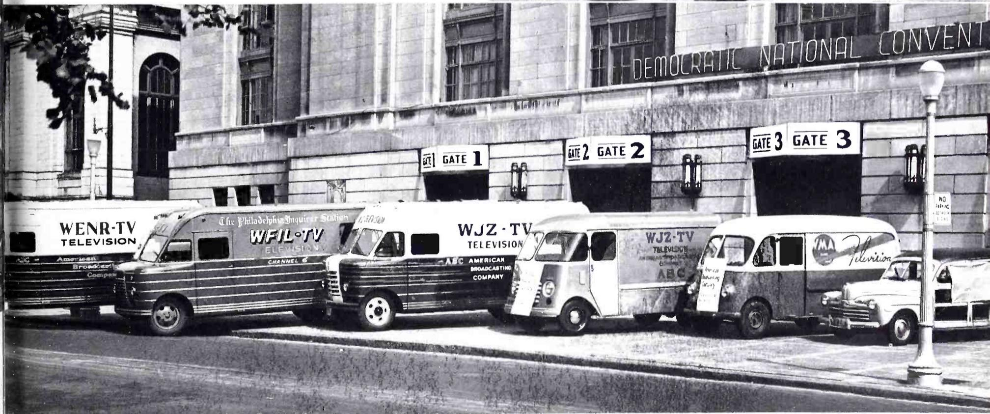
ABC's MOBILE UNITS lined up in front of Convention Hall give some impression of the way the networks made their plans to cover every activity associated with the Convention. The WENR-TV, WFIL-TV and WJZ-TV trucks are standard RCA TJ-50A Mobile Units. The smaller WJZ-TV truck is an auxiliary. Next to it is WMAL-TV's truck, and at the extreme right a station wagon equipped as an AM/FM mobile unit.
