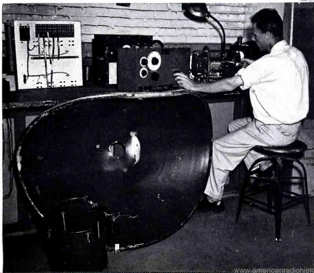
**SAME RECEIVER** after it was blown off of the 5 stories high roof by terrific storm. Parabola and can were badly twisted, and the latter had to be cut to remove chassis inside. However, when chassis was tested in RCA Laboratory (left) it was found to be still operative.
