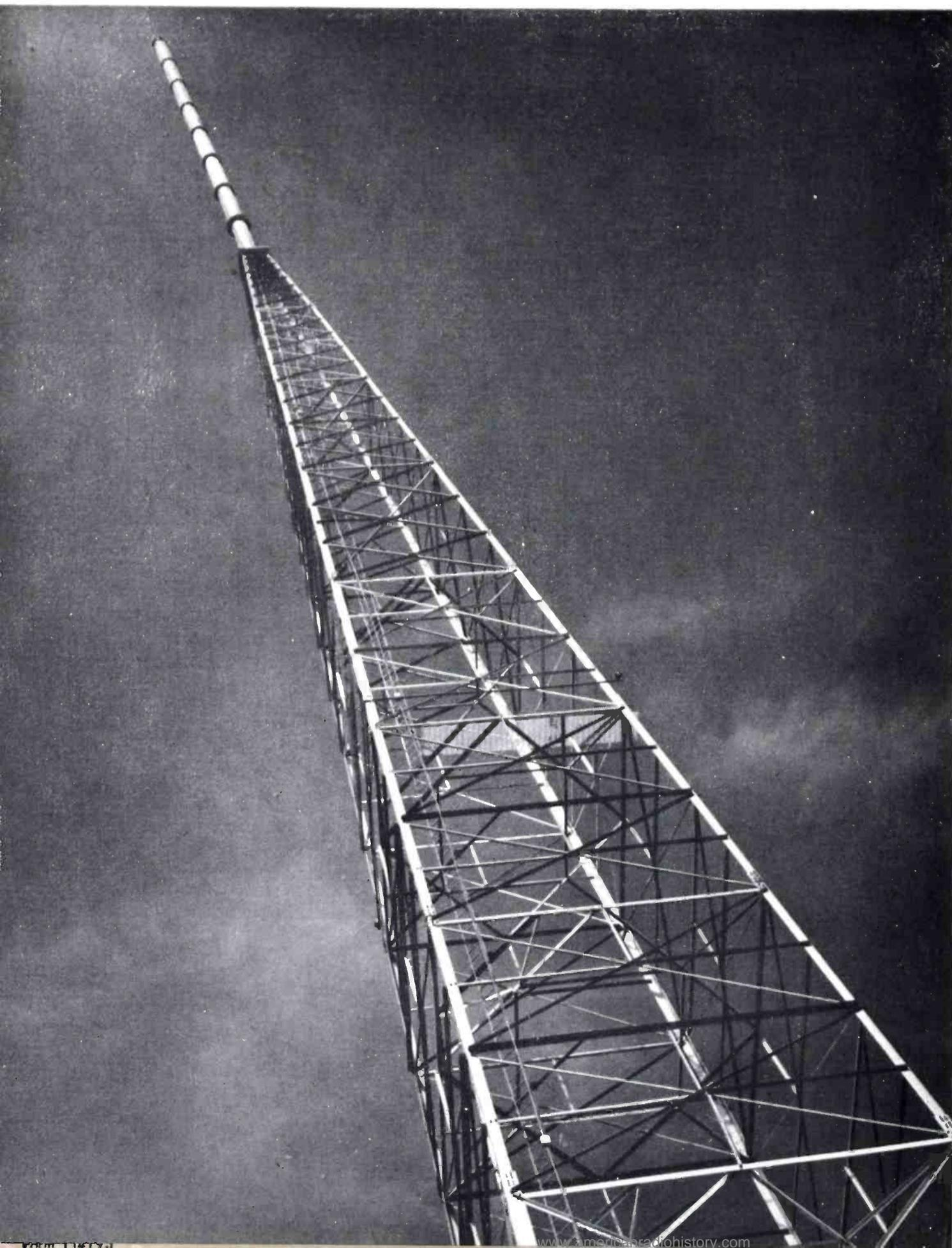
FIG. 1 (at left). Rising to a total height of 369 feet, the new "Super-Power" eight-section Pylon antenna provides an effective radiated power of 30 kilowatts.
