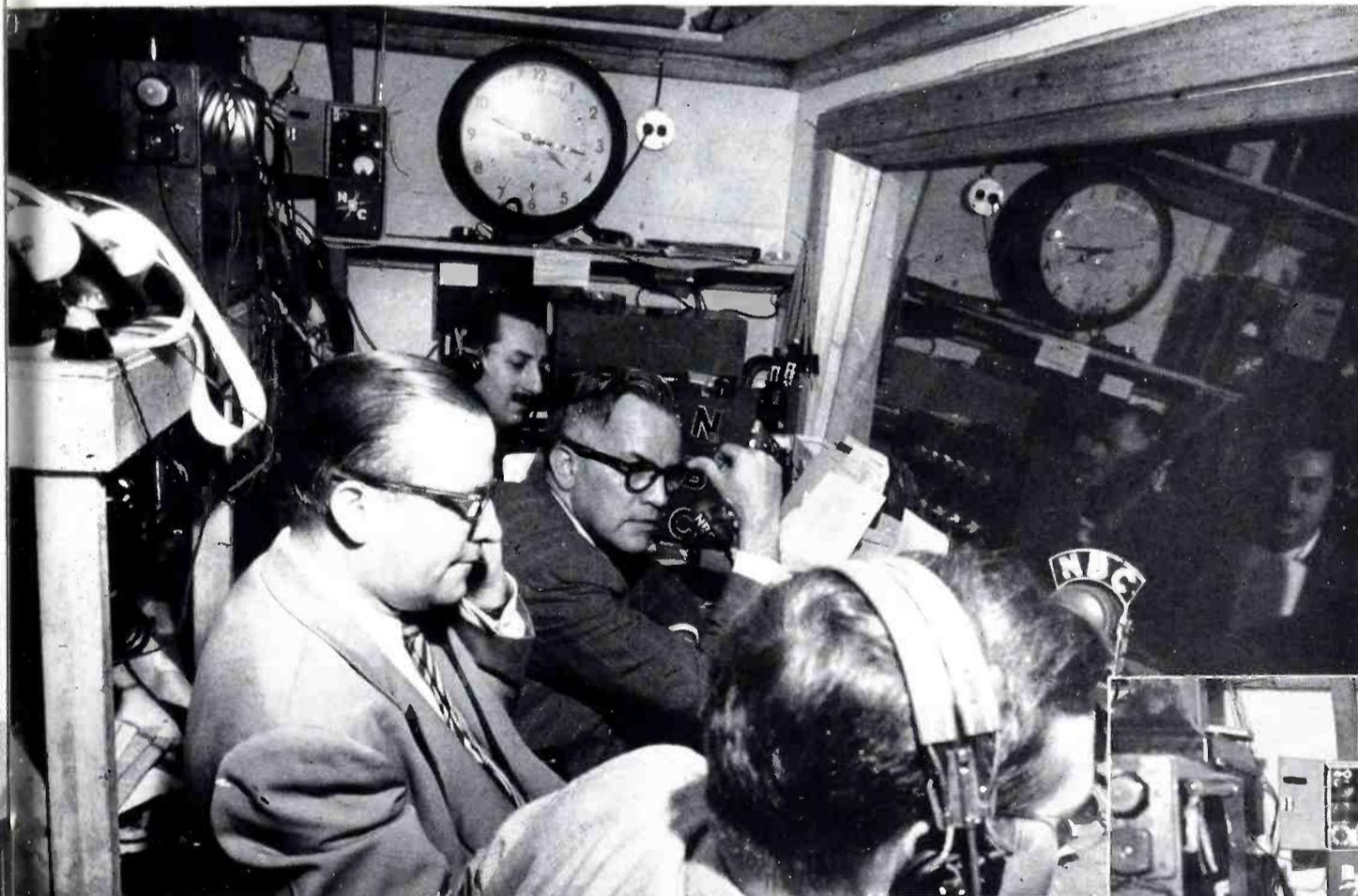
NBC's CONVENTION HALL AM/FM CONTROL BOOTH is shown above during actual operation. Announcers, analysts and news commentators sat along table in front of the window that looked out on the Convention Hall floor. Engineers position, at the far end in the view above, is shown closeup in the small illustration at the right. Portable equipment used by NBC are similar in general design to RCA OP-5A amplifier used by many stations.
