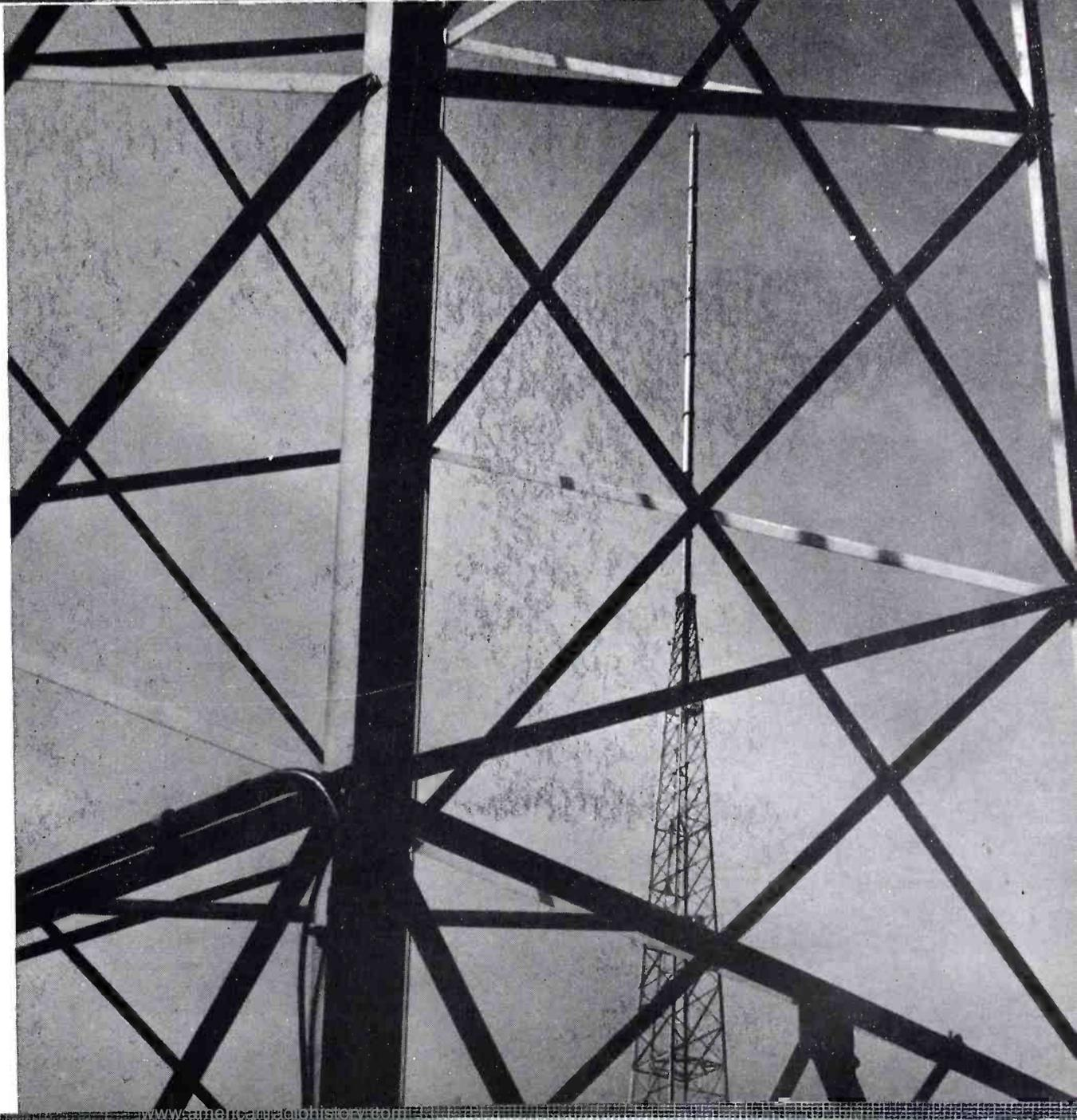
FIG. 3 (at right). Looking through one of the AM towers, the completely installed eight-section, high-power Pylon is visible.
