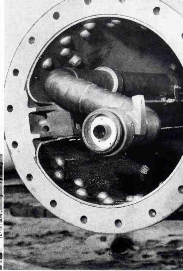
FIG. 12 (above). Closeup of the S-shaped crossover end of the transmission line for the top four sections, as it appeared during ground tests. The crossover connects to the feeder line running up the back of the bottom four sections. After ground tests, the S-shaped crossover was disconnected and tied inside the cylinder for safekeeping during erection.
