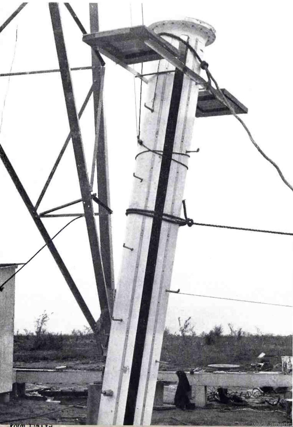
FIG. 8 (below). This view shows that three Pylon sections have been hoisted and mounted into place . . . and the fourth is on its way up the tower. Both tag lines and winch cables were controlled from one winch truck.
