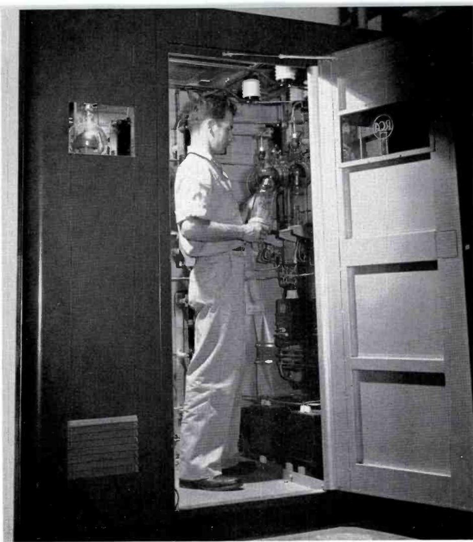
FIG. 9 (at left). WTMJ-FM engineer, Raymond Hernday, is shown installing an 857-B rectifier tube. This photo shows the "walk-in" type construction used for ease of operation and maintenance of all components of the 120 KVA rectifier unit. This rectifier supplies plate voltage to all power amplifier tubes down to and including the  $\frac{1}{4}$  KW amplifier.
