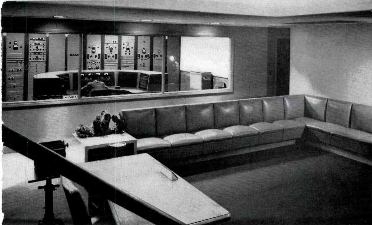
FIG. 3. This is just one of CMQ's modern waiting rooms. Adjacent to it is the master control room which is seen through the sound-proof glass partition. An operator is seated at the semi-circular master control console which monitors the network and local programs. Behind the console are located the numerous audio and test and measuring equipment racks.
