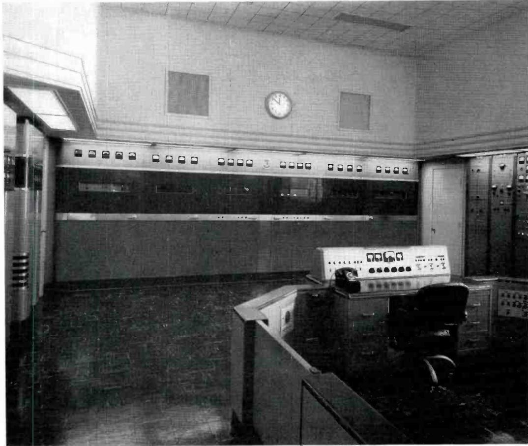
FIG. 2. The station is as neat looking inside as outside. Shown at right is the transmitter room which contains a 10 KW RCA Type BTA-10F Transmitter, a 1 KW BTA-1L Standby Transmitter, the speech input equipment, and the operator's control console.
