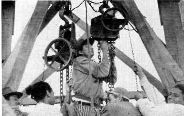
FIG. 23 (at left). Construction workers at the top of the Sao Paulo State Bank Building are shown during antenna "lifting" process.
