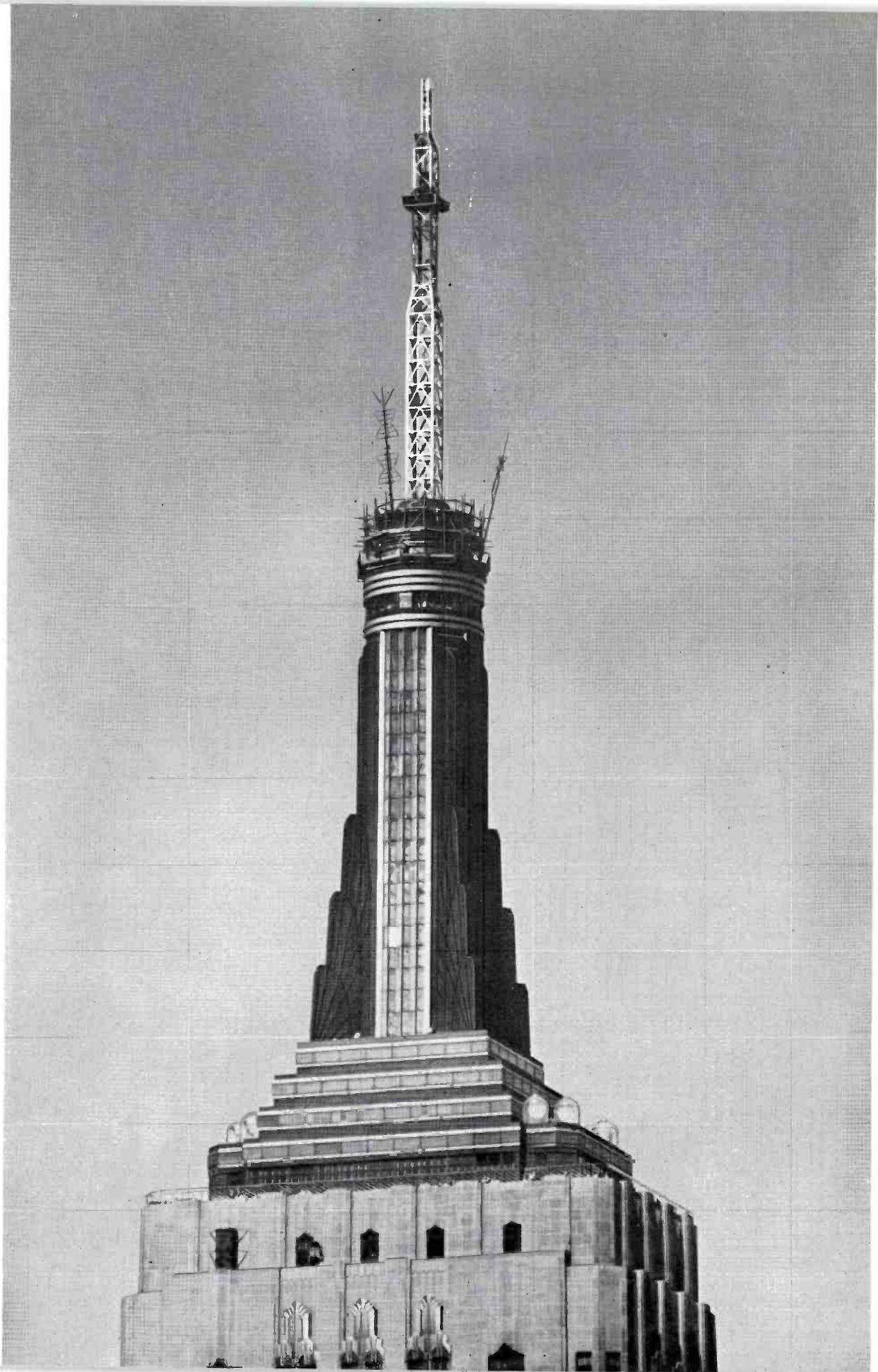
The 222-foot tower which will support five TV and three FM antennas 1472 feet above New York City is nearing completion. This photograph, taken with a telephoto lens, shows part of the third and last tower section to be erected. Completion of the tower will be followed by assembly of the Super Gain dipoles and screens around the four sides of the tower. A 4-section Super Turnstile will top the tower.
