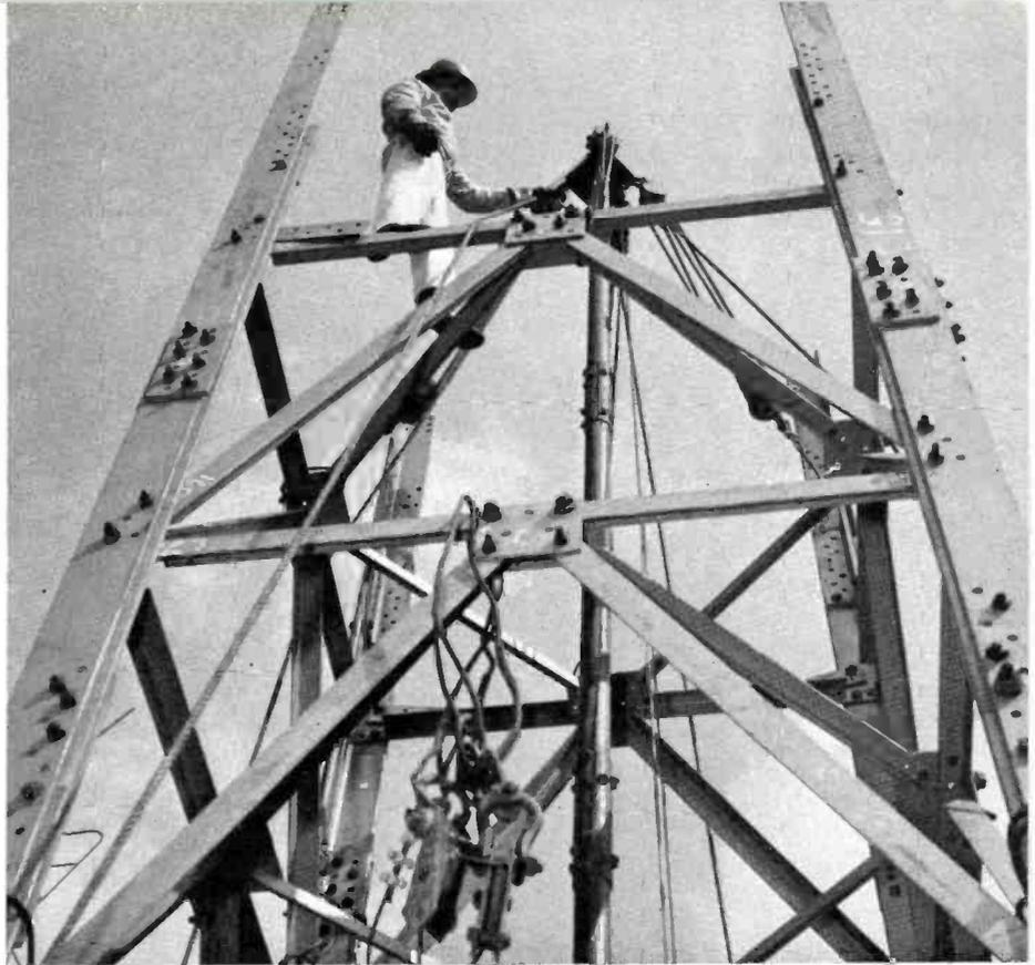
In raising the tower, steel sections are brought up inside the Empire State elevator shaft and then raised to position by block tackle on suspended gin pole shown at the top of tower.
