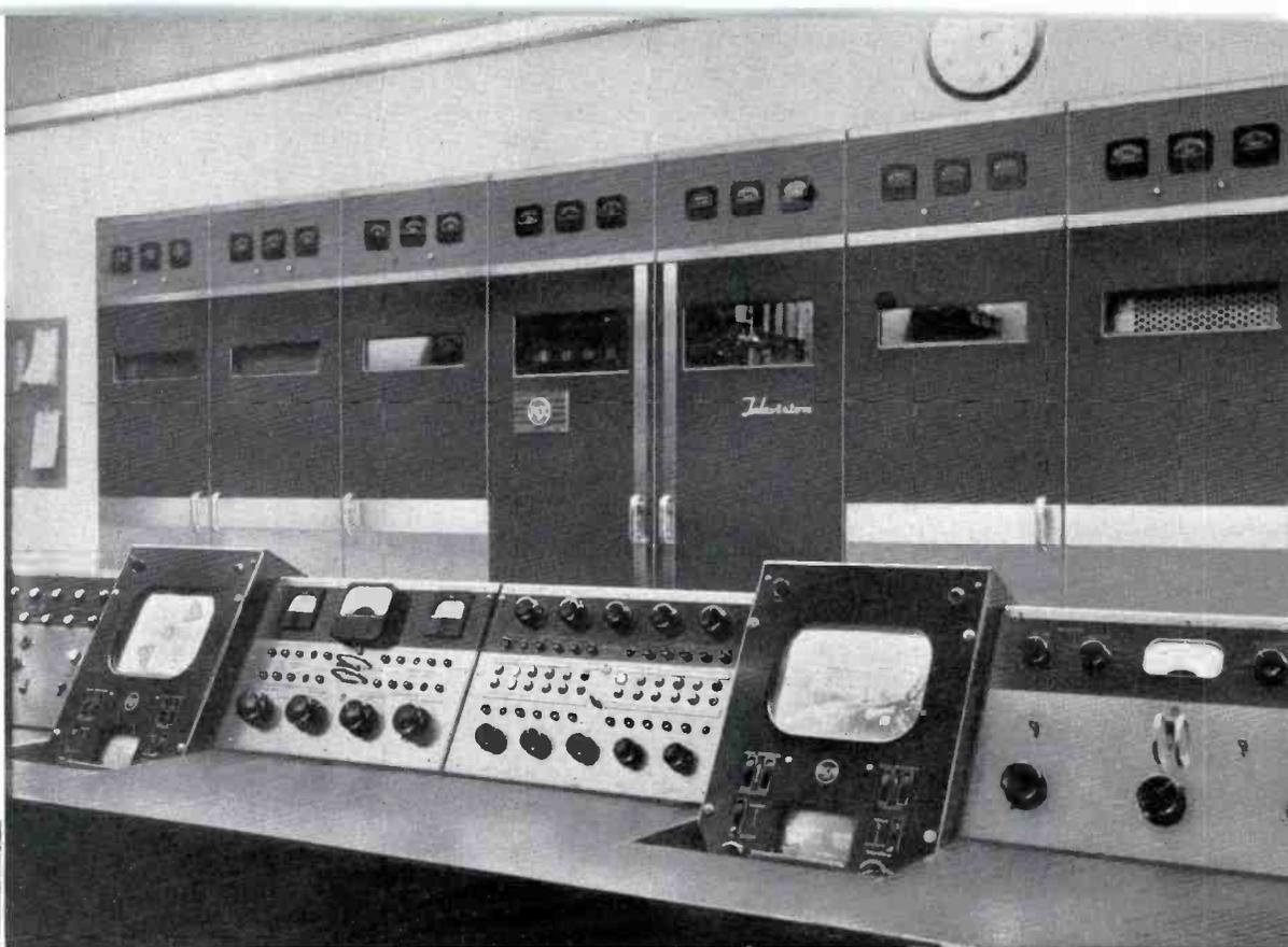
Photo above gives a better view of the FM-TV transmitter console, and TV program switching turret (center of photo). FM turret is at extreme right, TV transmitter monitor and control turrets at left. Right hand monitor unit is for program preview.
