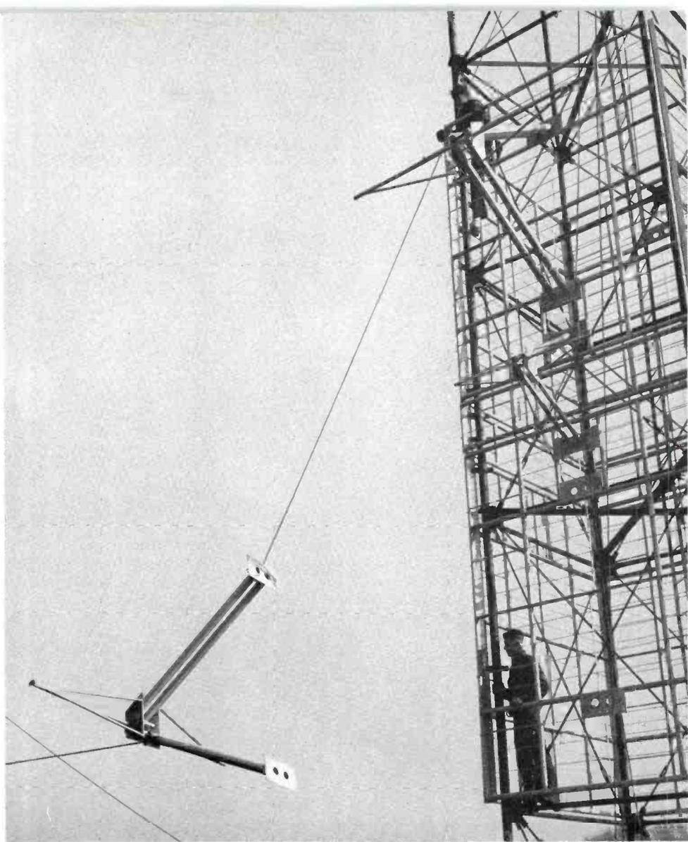
Channel 2 radiating elements being assembled on the screens prior to erection on the tower. Prefabrication of the screens and dipoles speeds erection.
