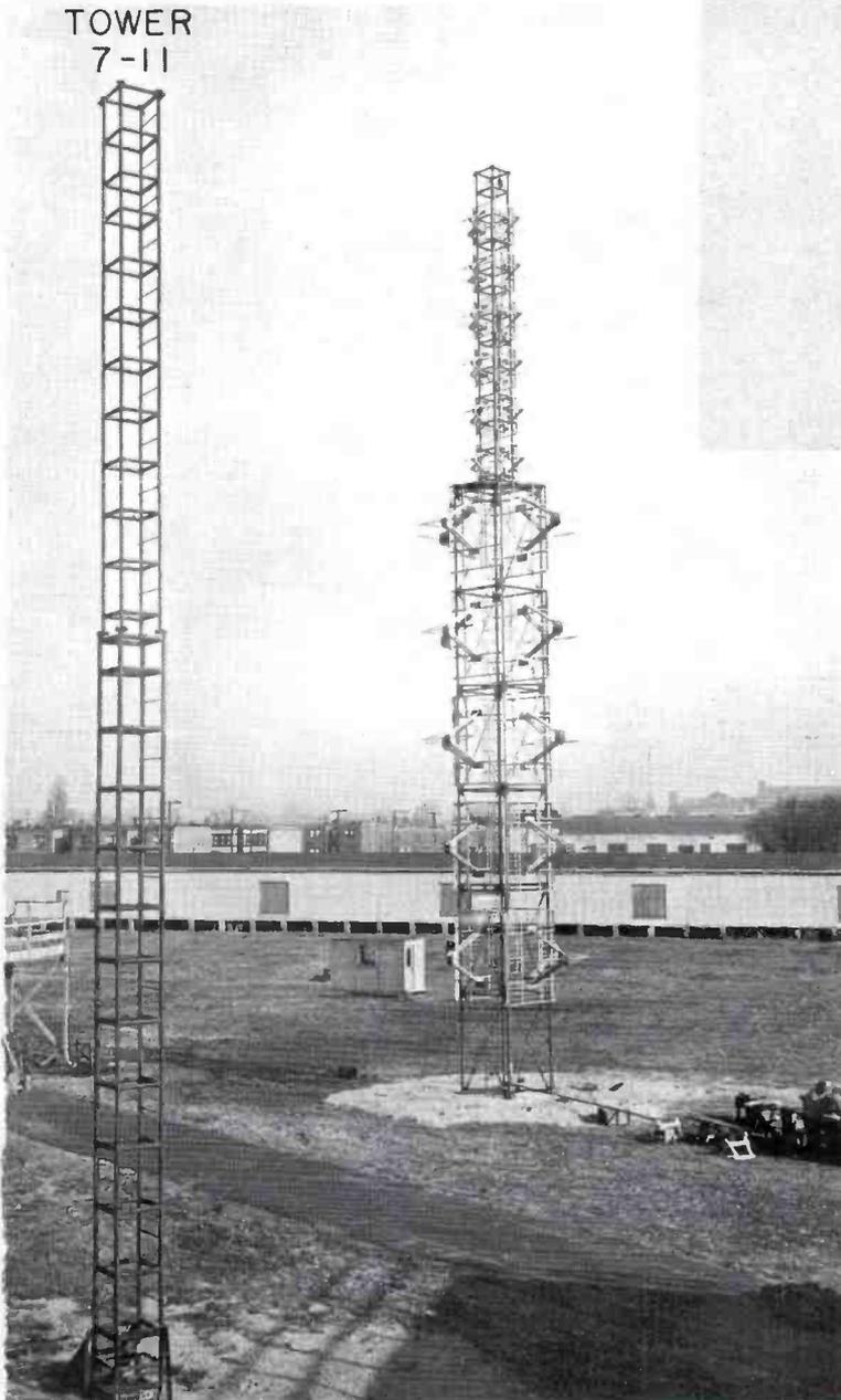
After tests have been completed on the 5-7 and 4-11 towers, the elements for Channels 7 and 11 will be moved to the 7-11 tower shown at left for further interaction tests. Installation of a wye in the transmission lines will permit feeding only part of the antenna for emergency operation.
