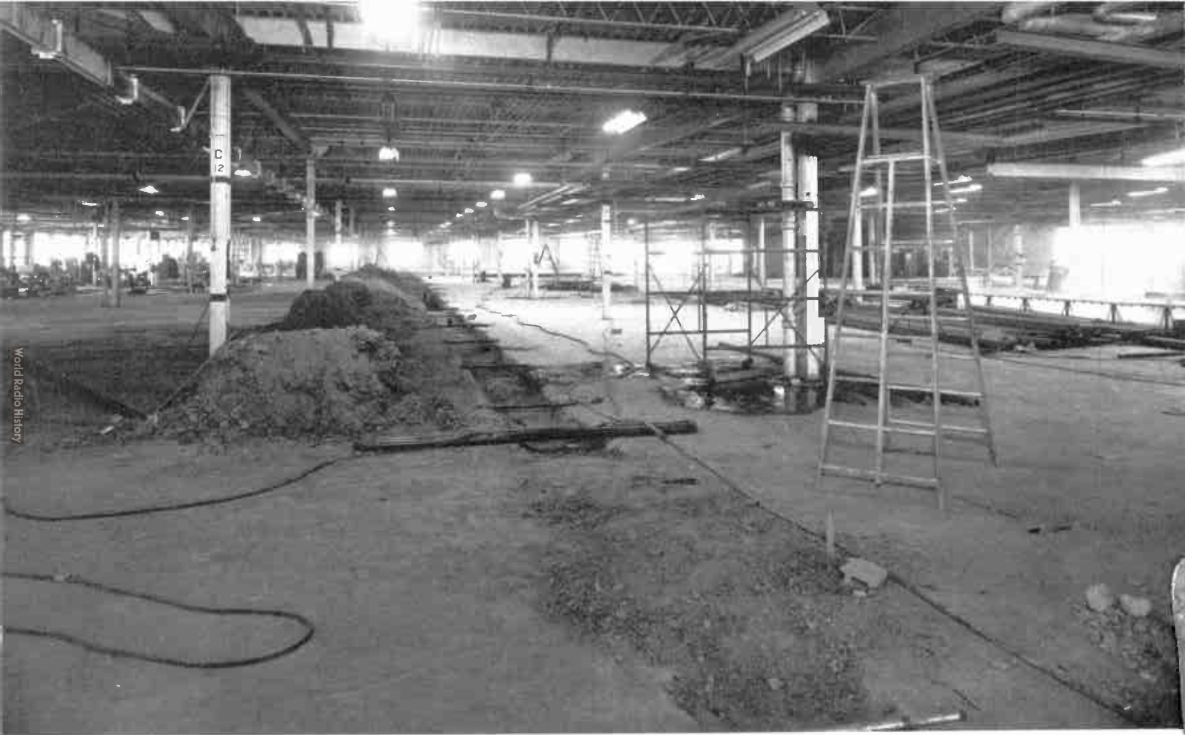
Sealex and mounting area in February
