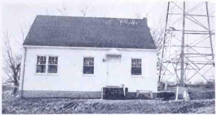
Fig. 3—Transmitter Building (front view).
