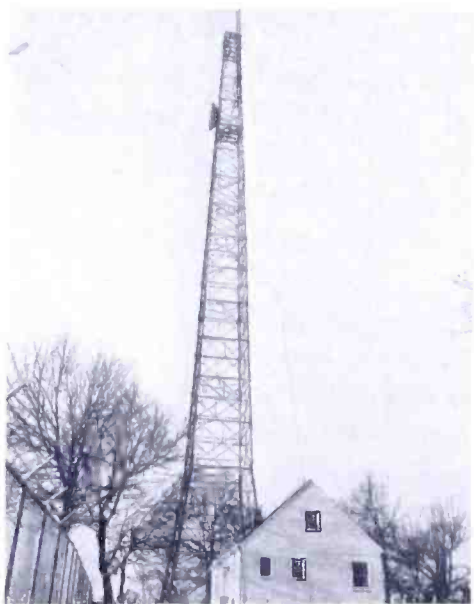
Fig. 6—Transmitter building (side view) and antenna tower. The Channel 4 parabolic receiving antenna can be seen at the 160 foot level of the tower.
