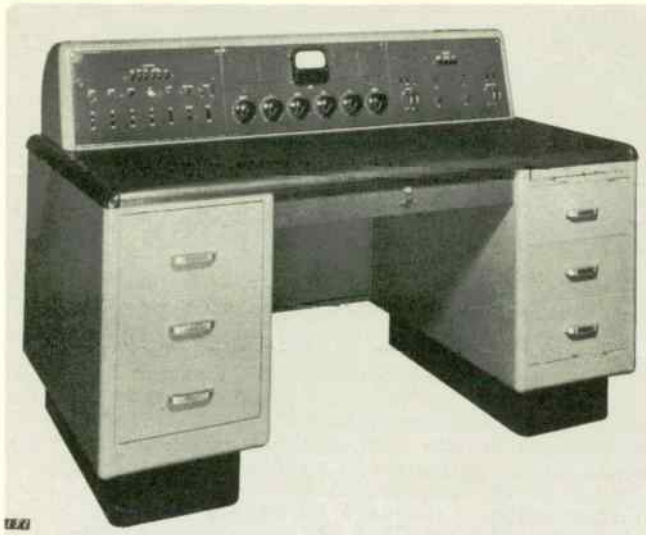
TRANSMITTER CONTROL DESK
