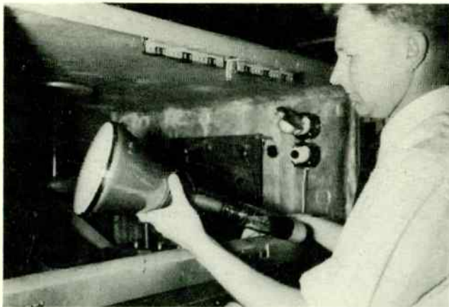
L. E. SWEDLUND PLACING 7-IN. PROJECTION KINESCOPE IN TEST COMPARTMENT
