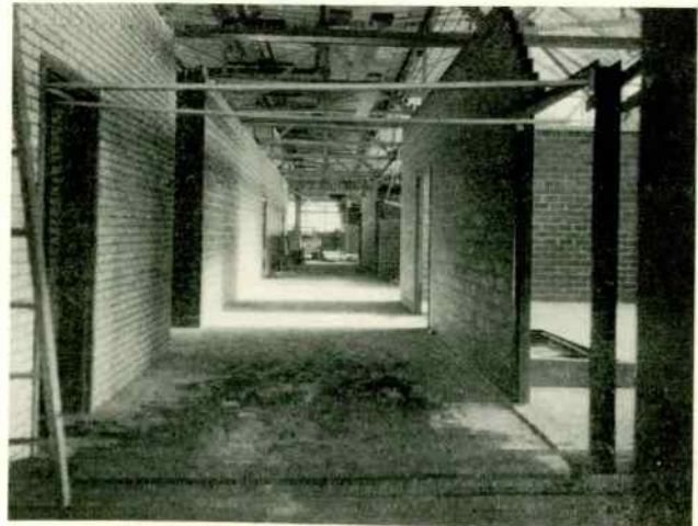
VIEW IN REAR BUILDING LOOKING SOUTHEAST DOWN CENTRAL HALL
