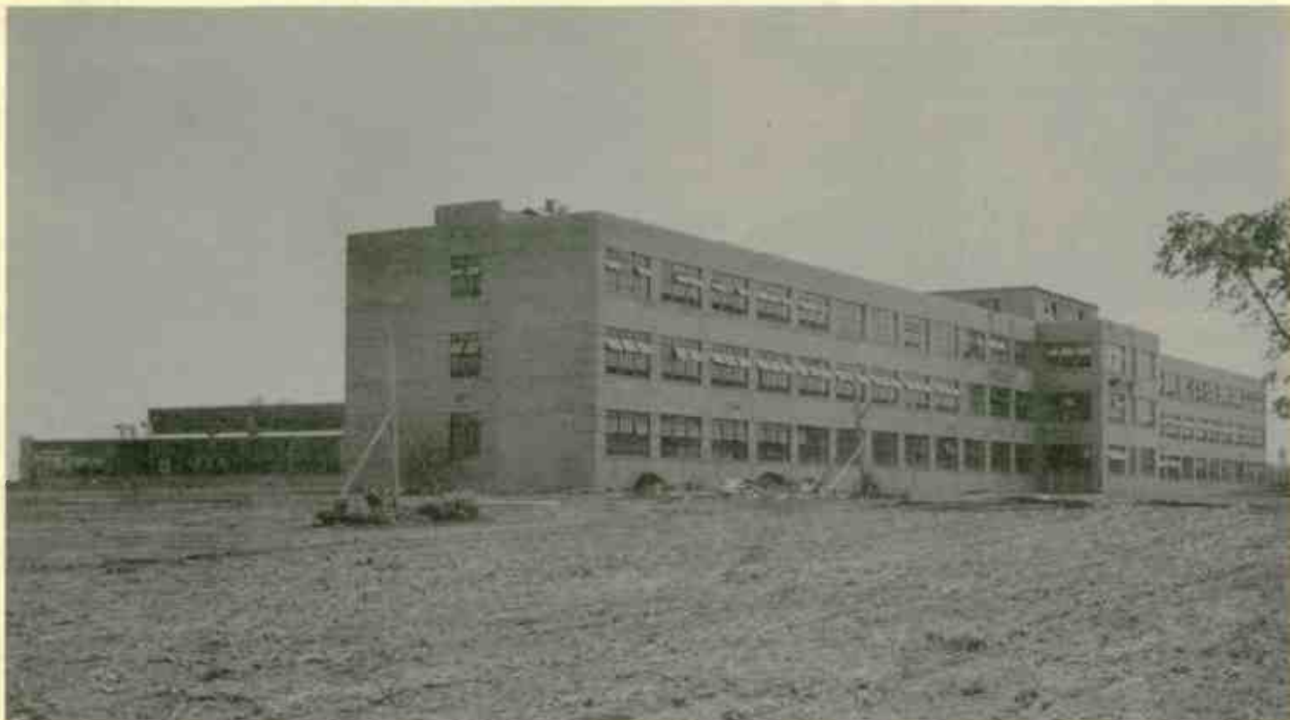
View of Main Laboratory Wing from the North
