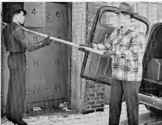
Bundled up warm, prior to tackling an installation on a cold Chicago day, are Jim Battiger, left, and Joe Cresham, right, installation men from Milwaukee Avenue.
