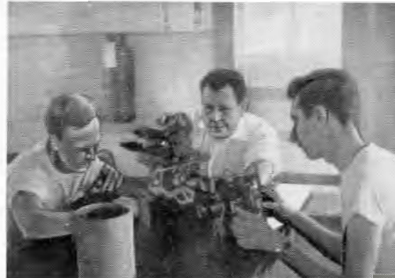
RCA techs in AF receiving station
