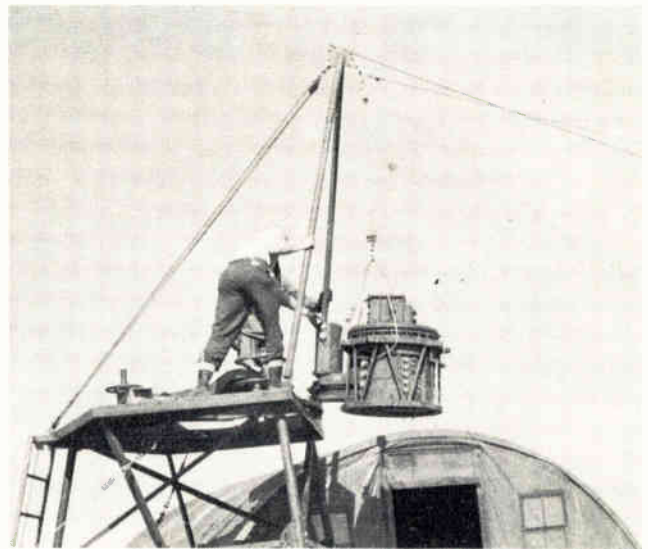
Harry working on equipment installation in Alaska
