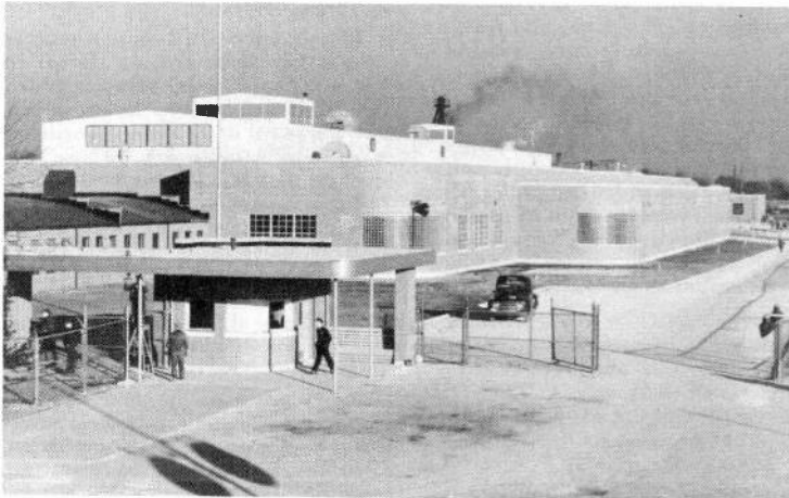
The RCA plant at Marion, Indiana which is being expanded to provide 50,000 square feet of additional space for the manufacture of tube parts.
