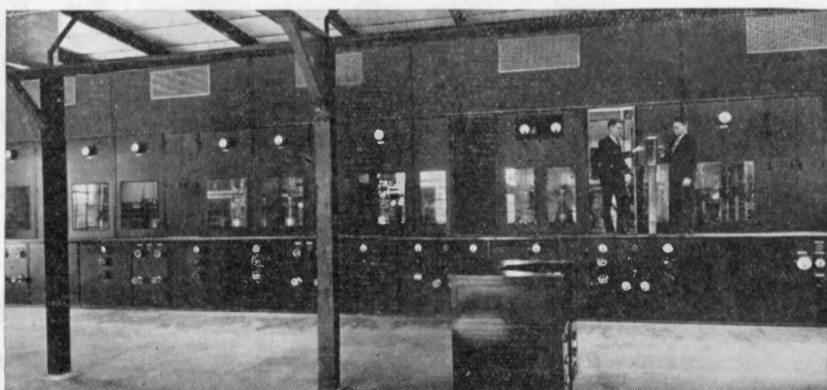
When Station WLW goes on the air, twenty 100-KW RCA Tubes supply the 500,000 watts that make WLW "the nation's station." Whether for giant broadcasting stations or home receivers, RCA Radio Tubes are standard.
