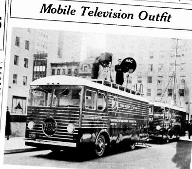
Typical of RCA's leadership in the development of television is this tele-vision transmitter caravan which will be used in New York in 1938. Note the iconoscope camera and antenna on the roofs of the cars. the iconoscope camera and antenna on the roots of the cars. This equipment will transmit by ultra-short wave to the Empire State Building atop which is the main transmitter used in RCA's television broadcasts
