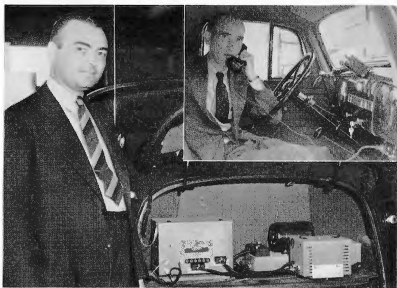
A. G. Kemp, RCA Victor representative at Cleveland, is shown at the left inspecting one of the city's new police cars equipped with two-way RCA Police Radio. The upper right shows Lloyd Chatterton, Superintendent of communication of the Cleveland Police Department testing one of the new installations by talking back to headquarters
