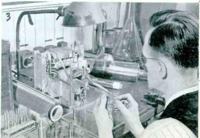
(3) Building an electron gun is a meticulous job for it is a delicate, yet powerful element in the "eye" of the television camera and receiver.
