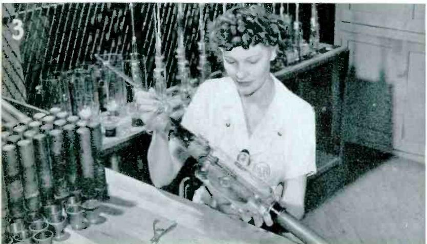
(3) By replacing worn-out elements, skilled RCA workers instituted an extensive program for reclaiming radio tubes for the war effort.
