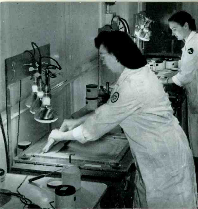
Preparing phosphor screen for RCA color TV picture tubes.
