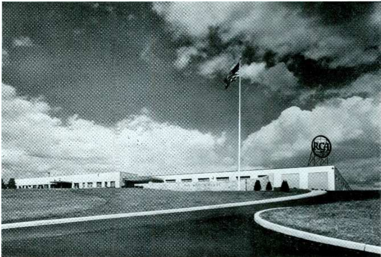
Modern manufacturing plant of the RCA Victor Division in Cincinnati where highly developed automatic machines produce miniature and sub-miniature tubes for radio and television.
