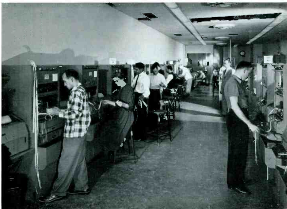
Most RCA radiotelegrams are channeled through "package sets" like these in traffic room at RCA Communications' San Francisco office.
