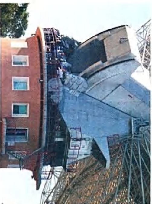
Brett Davison VK3CDBD repairing the hanging cable network, which allows the dish to rotate 540 degrees before needing to unwind. Brett, the Receiver Engineer and second in charge at the facility, explains that the cable run is 150 metres from the analogue receiver units on the third level of the building up to the Focus Box. VK3KRB
