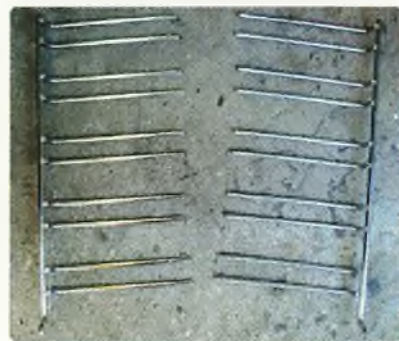
Photo 1: Cable rack cut.
