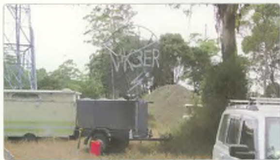
Photo 4: Peter VK3QI needed some markers to assemble the dish and the calsign is his way of assembling the pieces in the correct position.
