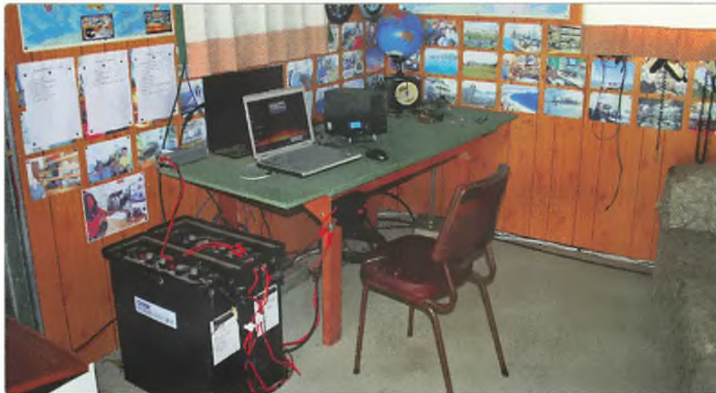
Photo 2: The remote station which is solar powered.
