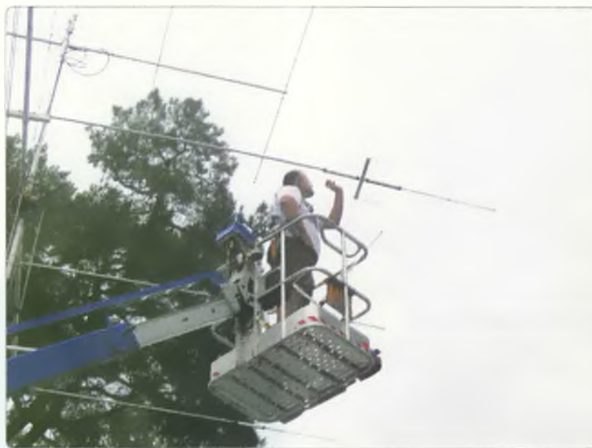
Photo 1: Jamie Giddons from Access Hire installing the 40 m traps on the HARG HF Beam.
