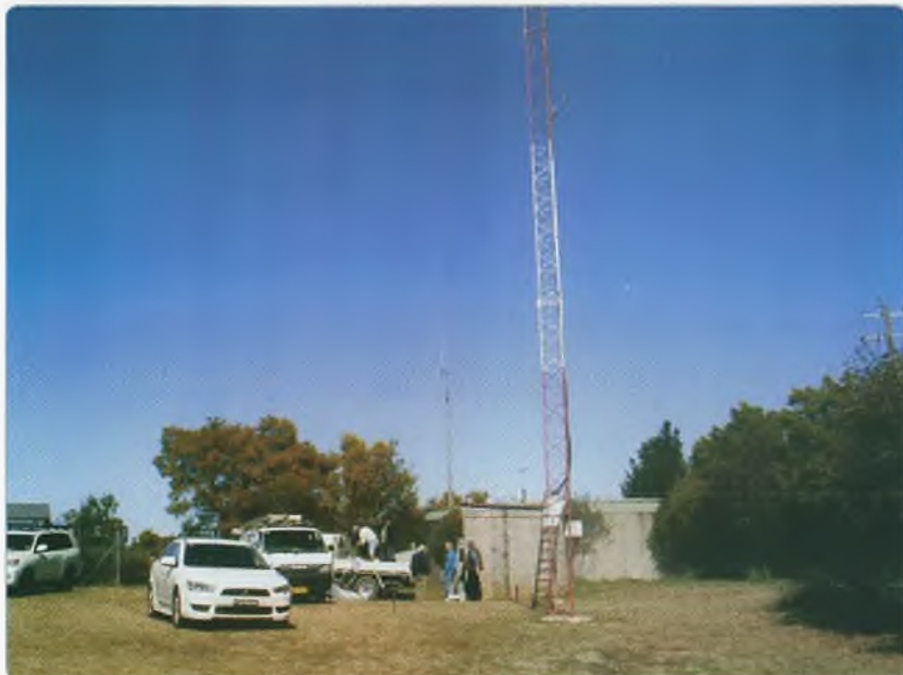
Photo 2: External view of the tower and hut.
