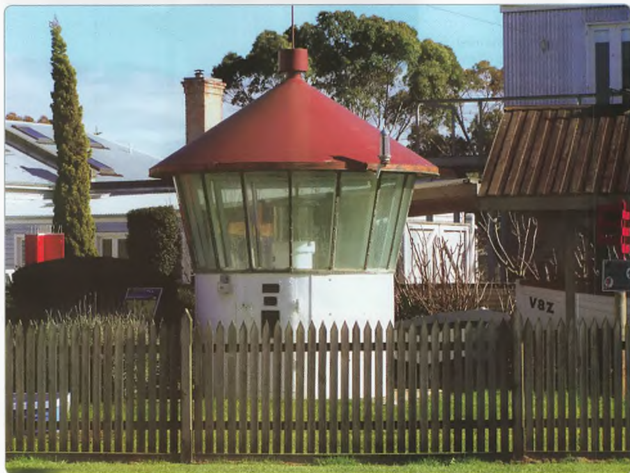
Photo 1: The top of the old Citadel Island Lighthouse.
