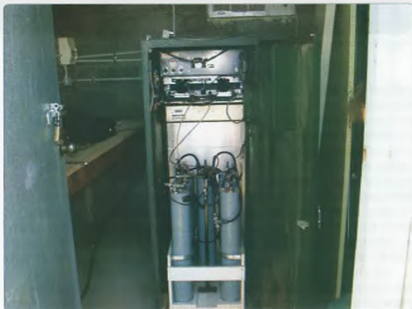
Photo 3: View of the repeater internals.
