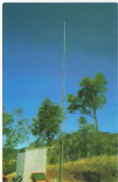
Photo 2: The CQARA 70 cm repeater mast and antenna at Bouldacombe, near Rockhampton. Output is 30 watts. EchoLink Node 9003.
