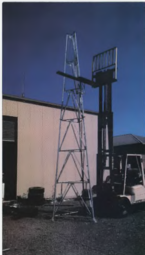
Photo 2: The new freshly galvanized replacement VK7RMD tower ready to airlift into place. Photo courtesy of Dion VK7DB.
