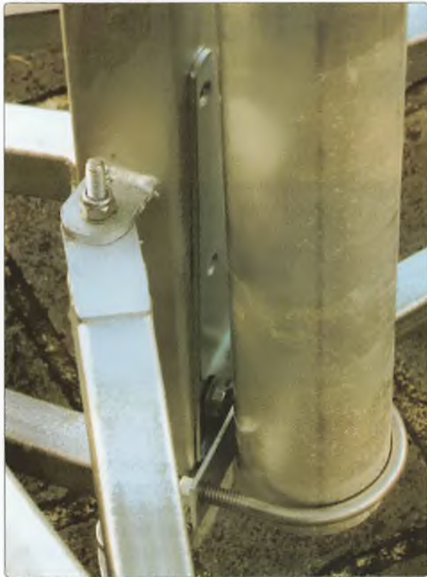
Photo 8: The hinge secured to the upright.
