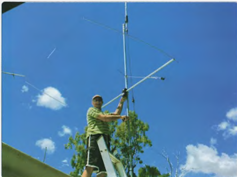
Photo 2: Ray VK4HOT working on the Par Electronics 20 metre Omniangle antenna at Weasel Park.
