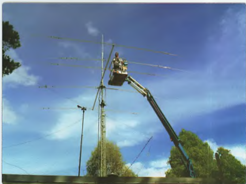
Photo 1: The HARG dipole installation, courtesy of Jamie's cherry picker.
