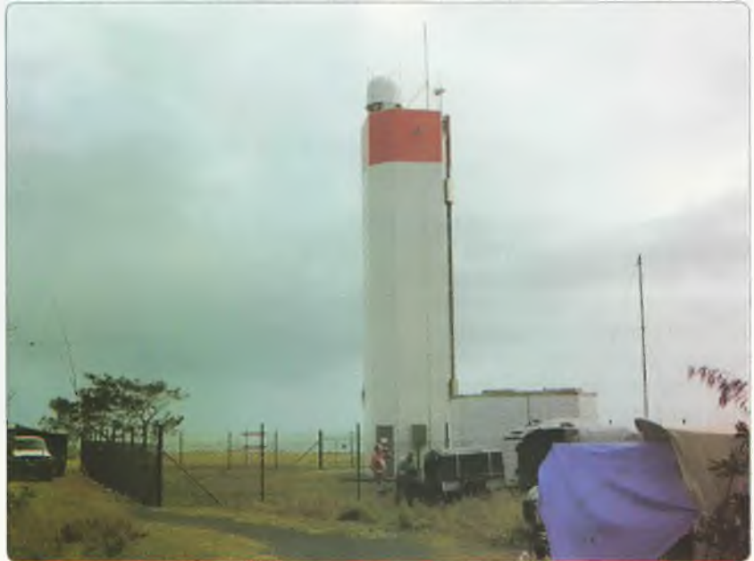
Photo 1: New Burnet Heads lighthouse.
