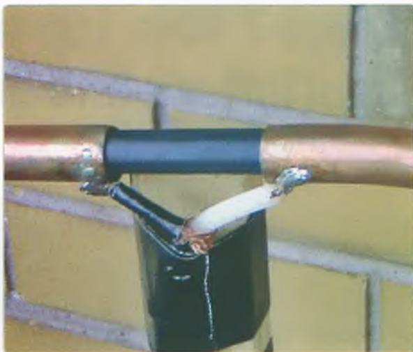
Photo 2: Coax cable capacitor soldered across top of loop.
