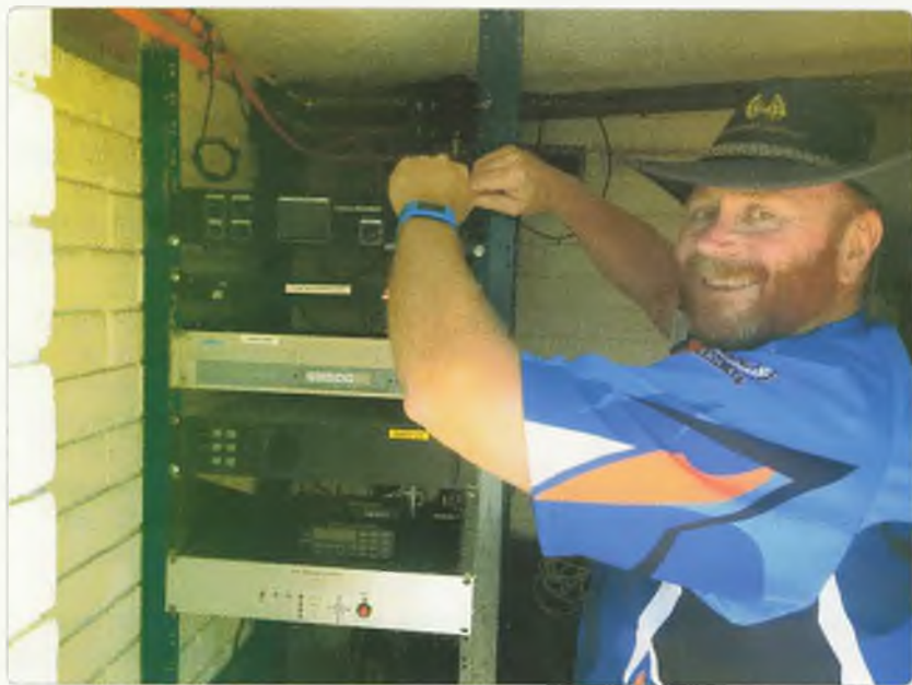
Photo 1: Ray VK6ZRW installing the Yaesu Fusion repeater.
