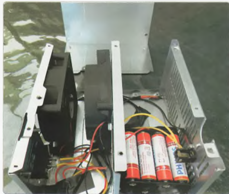
Photo 2: Interior view showing layout.
