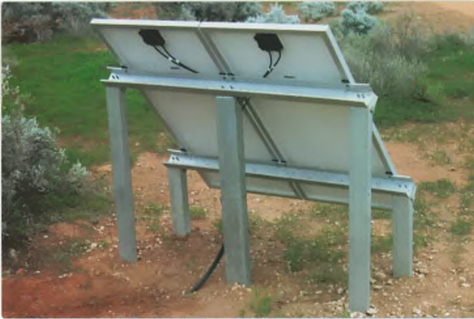
Photo 7: The purpose built galvanised steel frame.
