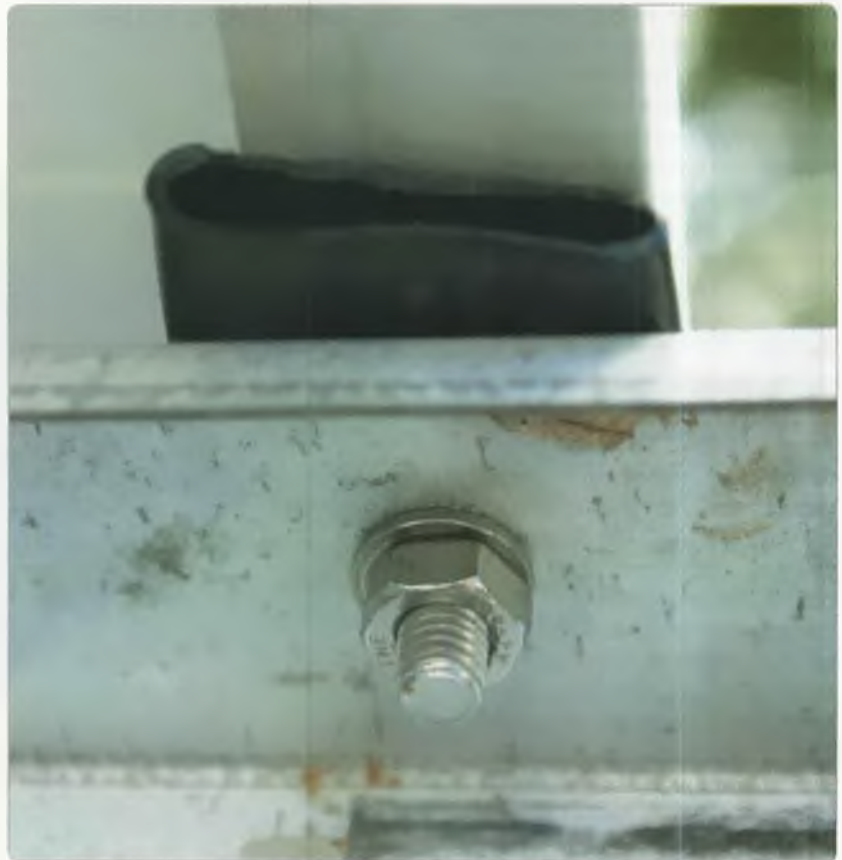
Photo 8: The plastic irrigation hose insulator.
