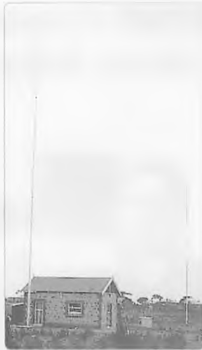
Photo 4: 5MU Building & its original 100 ft masts with tuning hut.
