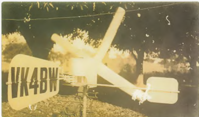
Photo 7: Home made wind generator mid 1930s. (WIA Archive).
