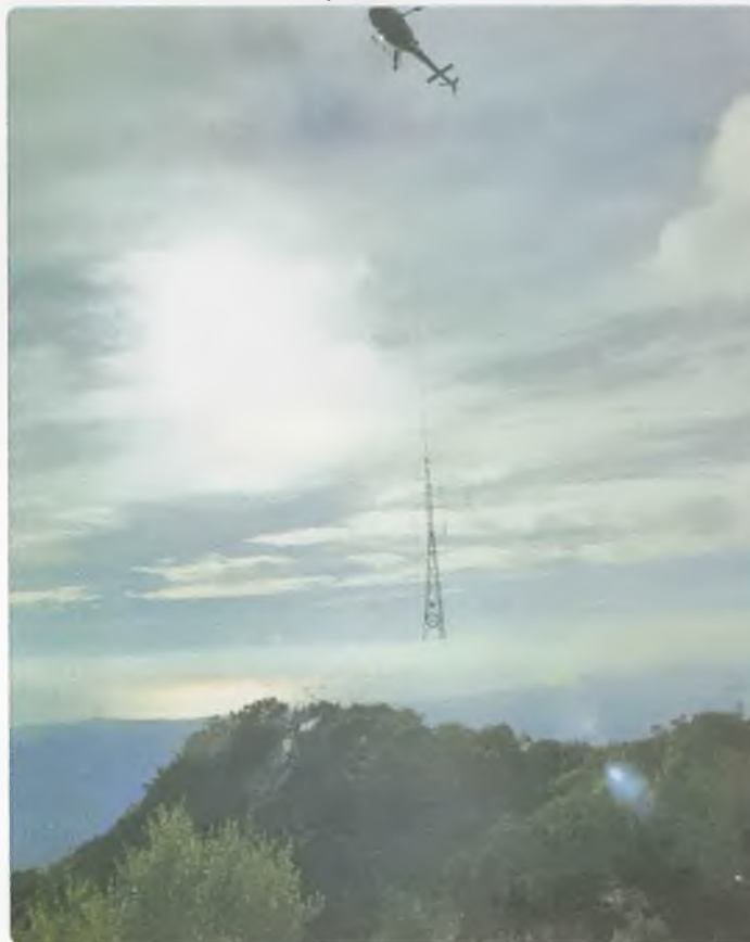
Photo 6: The tower almost in position.
