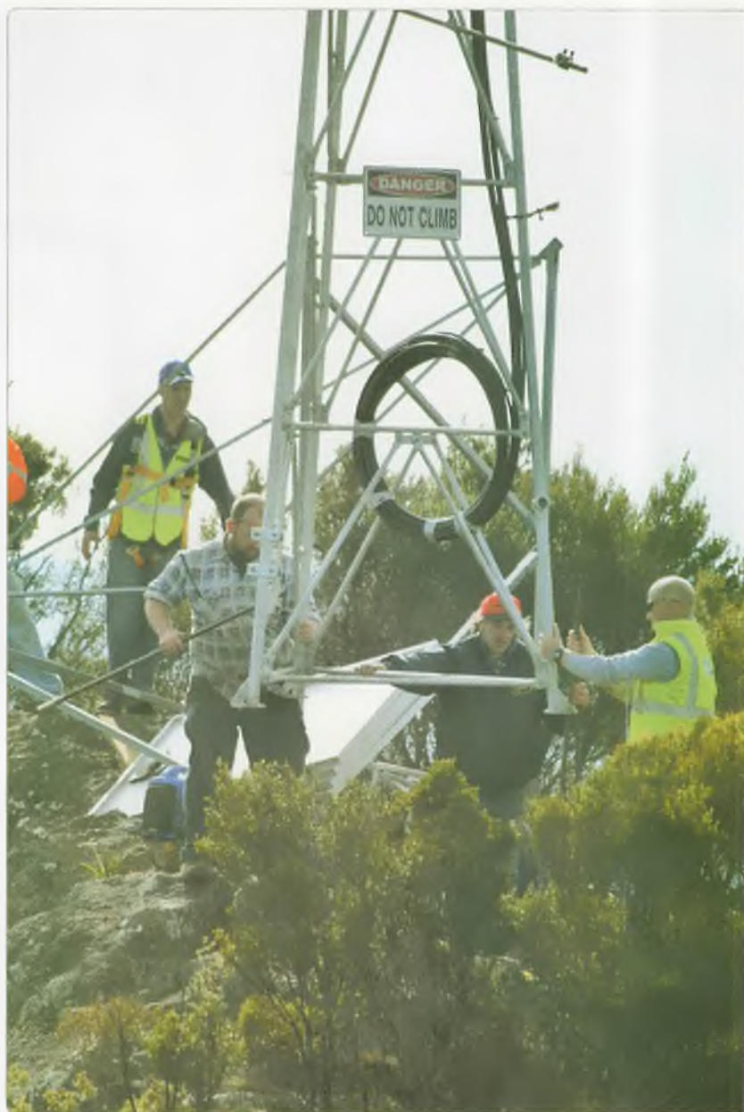
Photo 7: Tower guided in.
