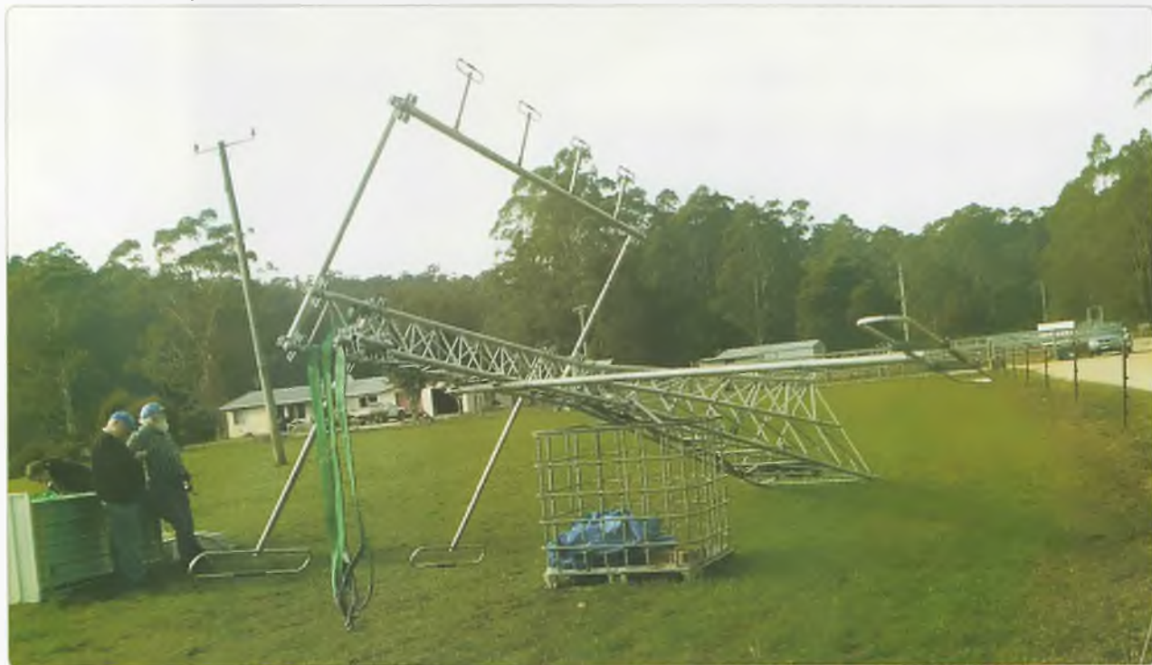
Photo 2: Tower ready to lift.
