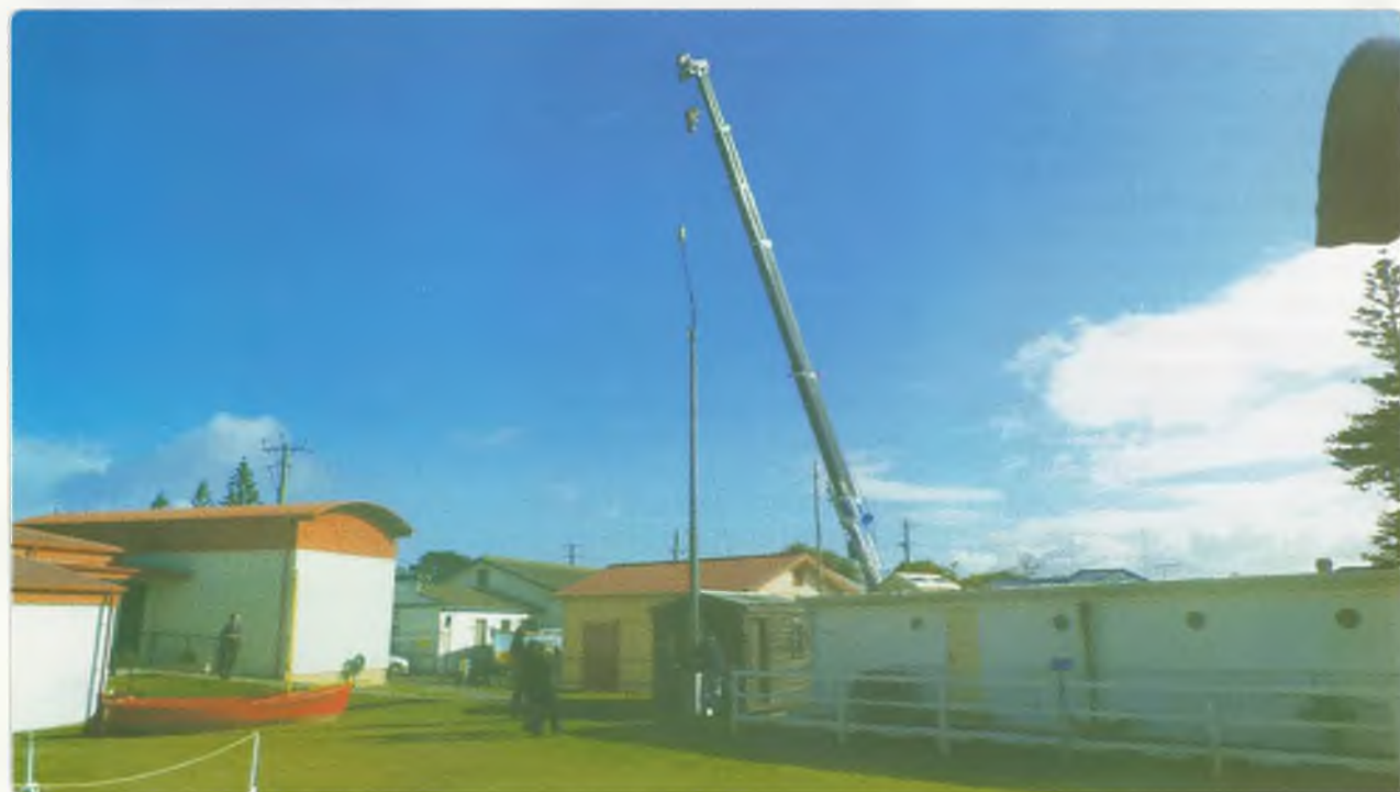
Photo 1: Installation of the mast.
