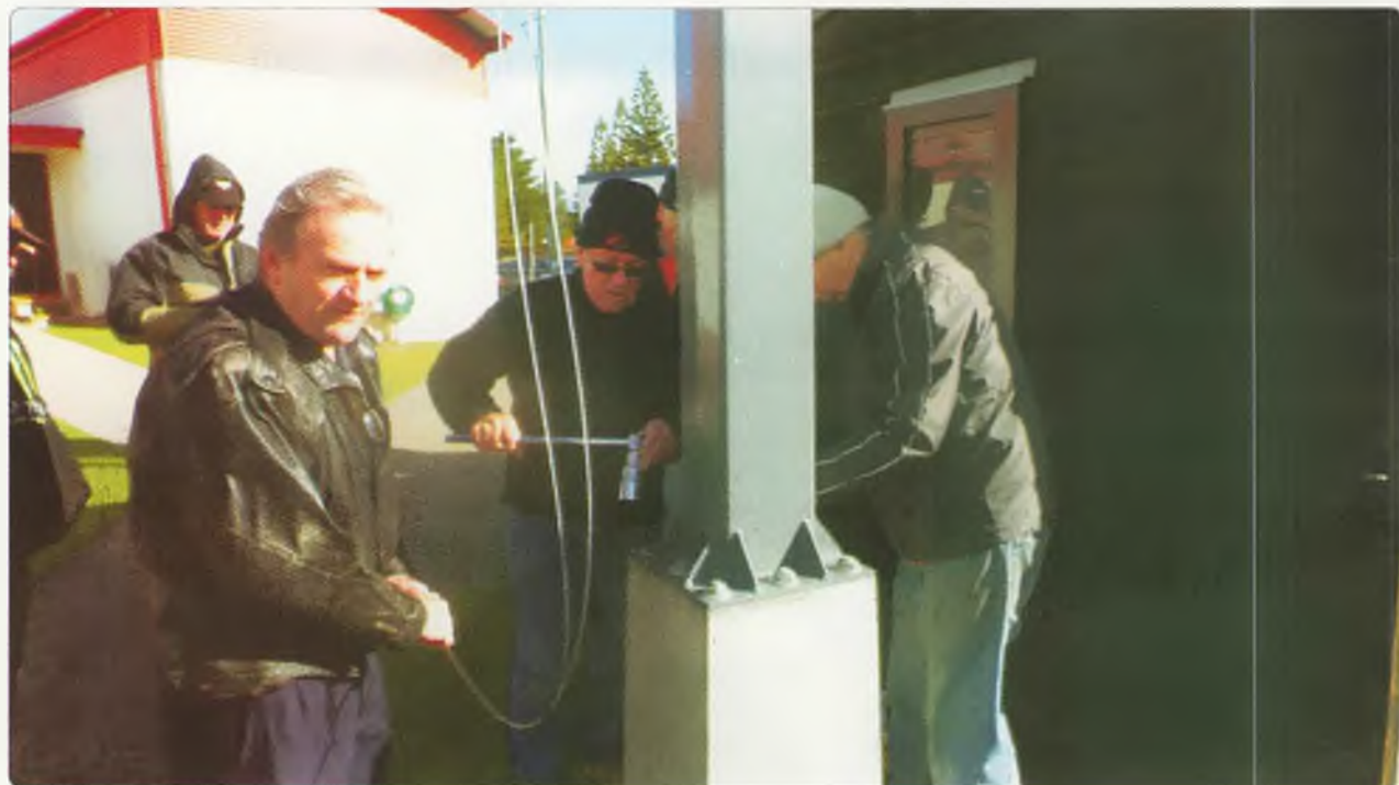
Photo 2: Bolting the mast to the mounting base.
