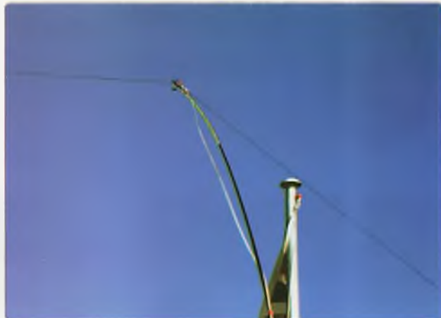
Photo 3: Feedpoint at dipole.
