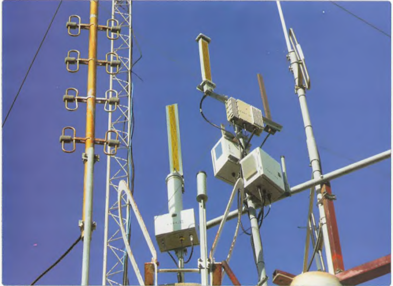
Photo 1: The five beacons installed on the Water tower: three enclosures near the centre are the 3.4, 5.7 and 10 GHz units. The enclosure below and to the left of centre houses the 1.2 and 2.4 GHz beacons.
