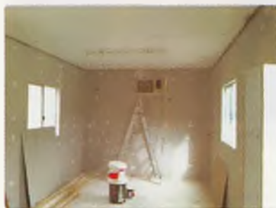
Photo 2: The interior after re-sheeting.
