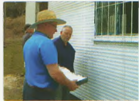
Photo 3: Norm VK4ANB and Les VK4FAEB putting the second coat of white over the original blue.
