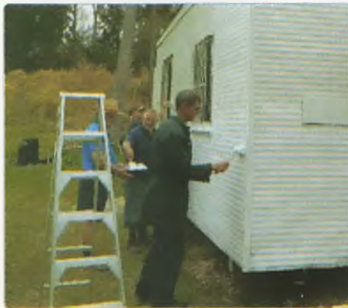
Photo 2: Working Bee team applying paint.
