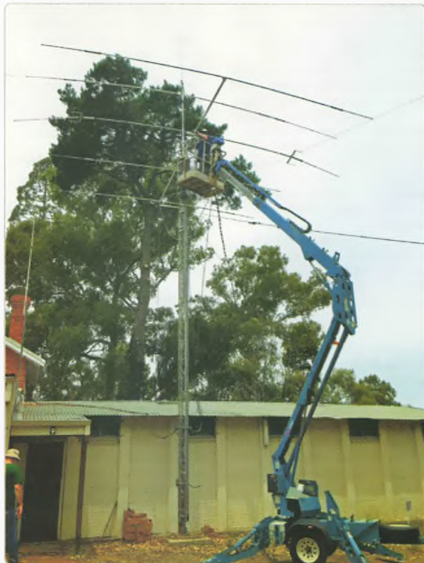
Photo 1: John VK6AG repairing traps on the HARG beam. Photo by VK6ZMS.
