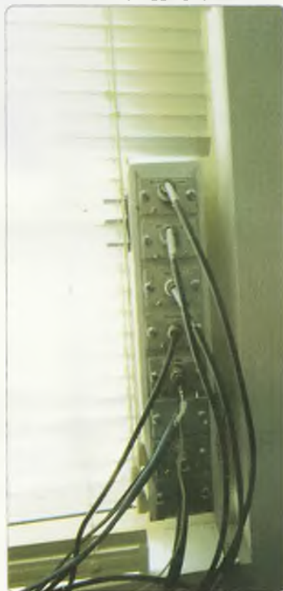
Photo 2: Vertical plugging system.
