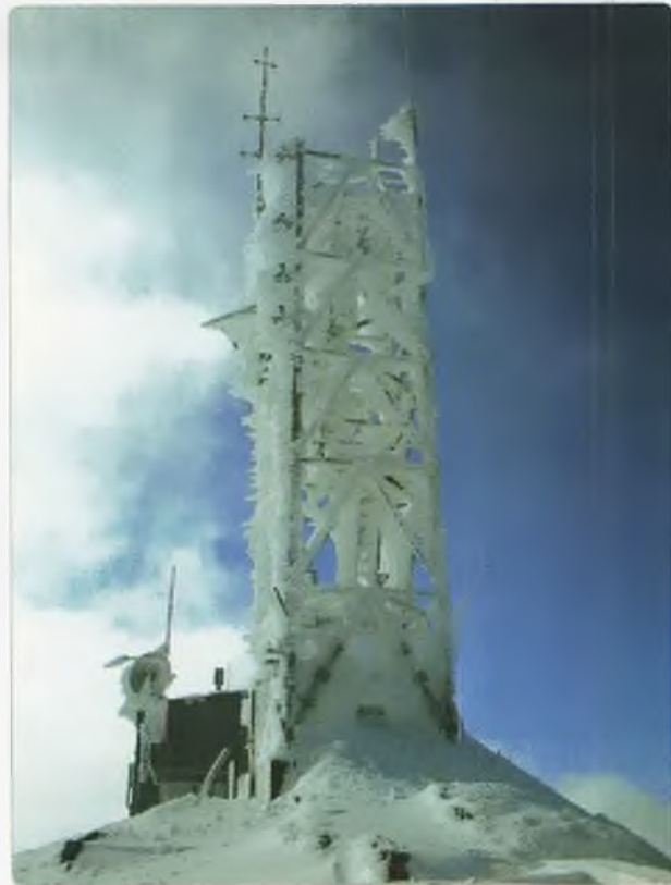
Photo 4: The summit communications tower encrusted with snow and ice.
