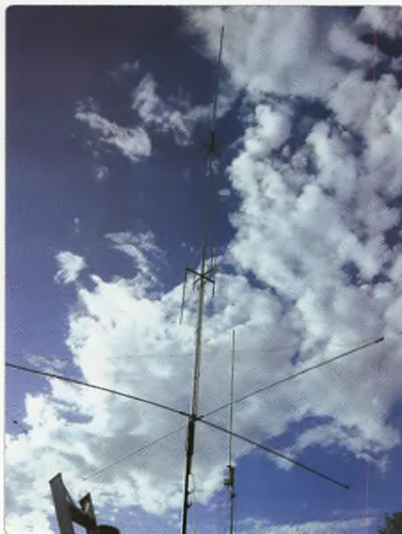
Photo 4: The antenna in the air ready for initial testing.
