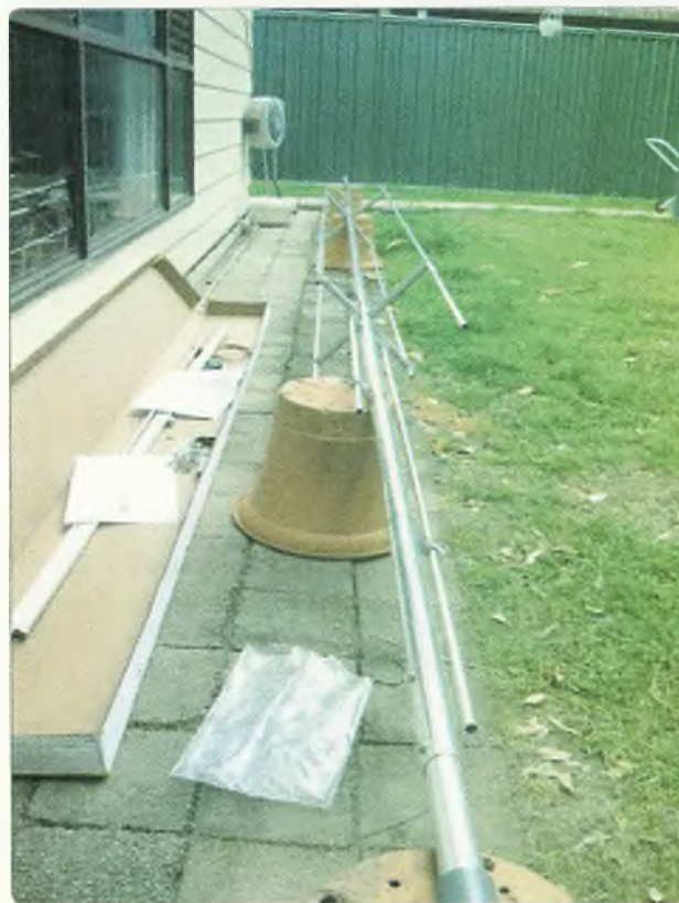
Photo 3: Assembly is progressing well.
