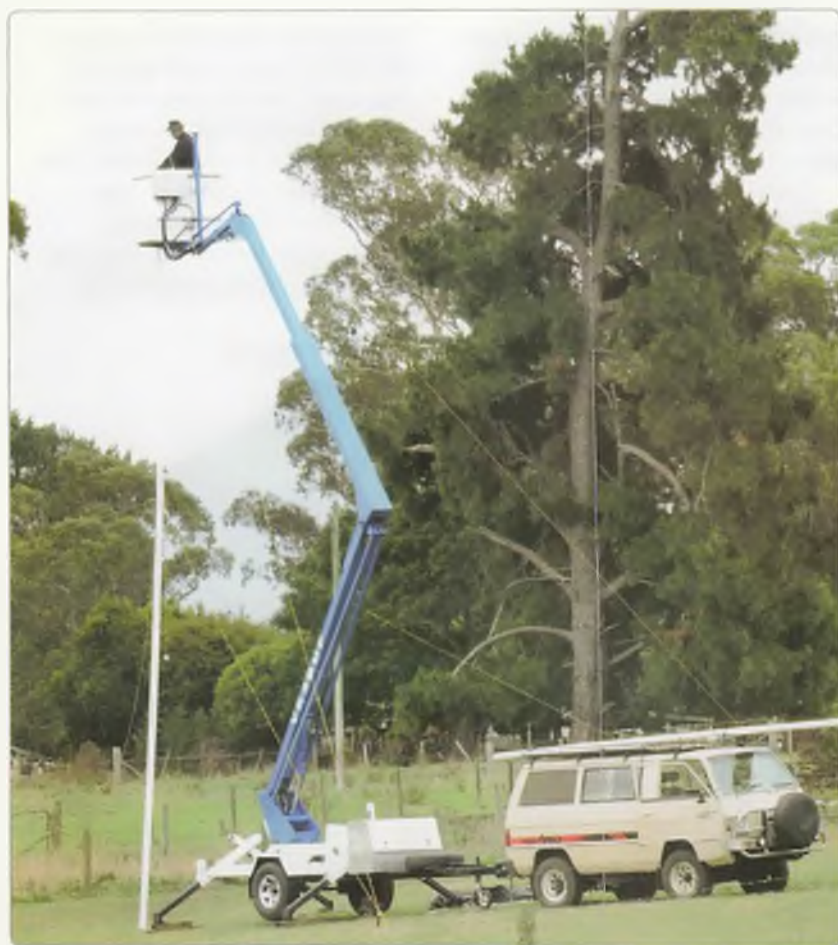
Photo 4: Ian VK3BUF preparing the 12 metre antenna poles for the rhombic.
