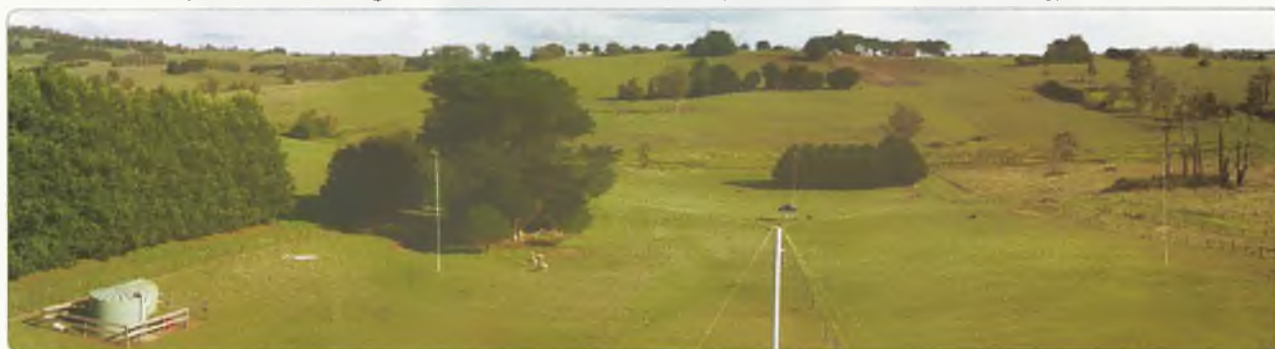
Photo 5: The completed 12 metre high rhombic antenna on 40 metres (wire radiator enhanced for clarity).
