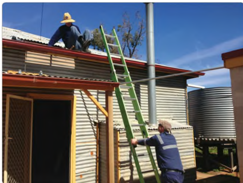
Photo 1: Jim Haywood on the roof with James VK2FDAQ holding the ladder.
