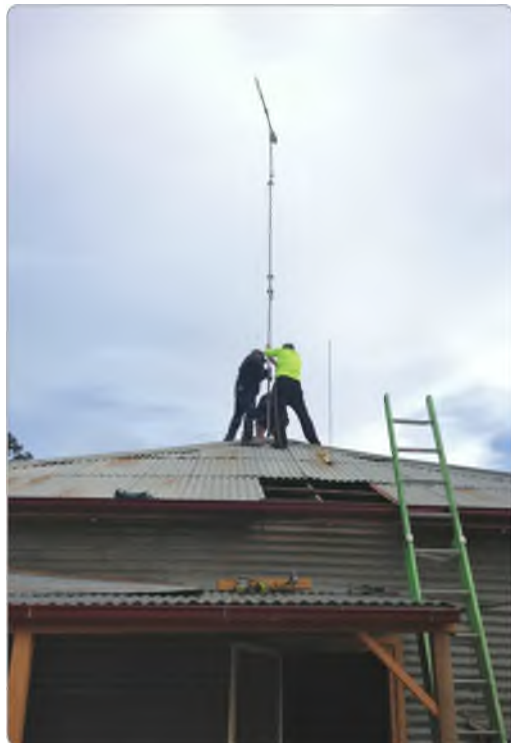
Photo 2: Installing a mobile phone antenna in the Murray-Sunset National Park.
