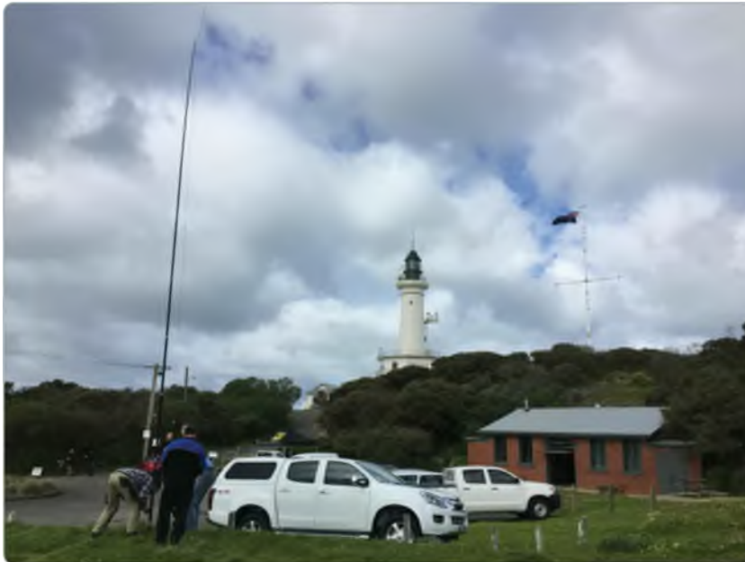
Photo 1: Antenna erection at the Lighthouse.
