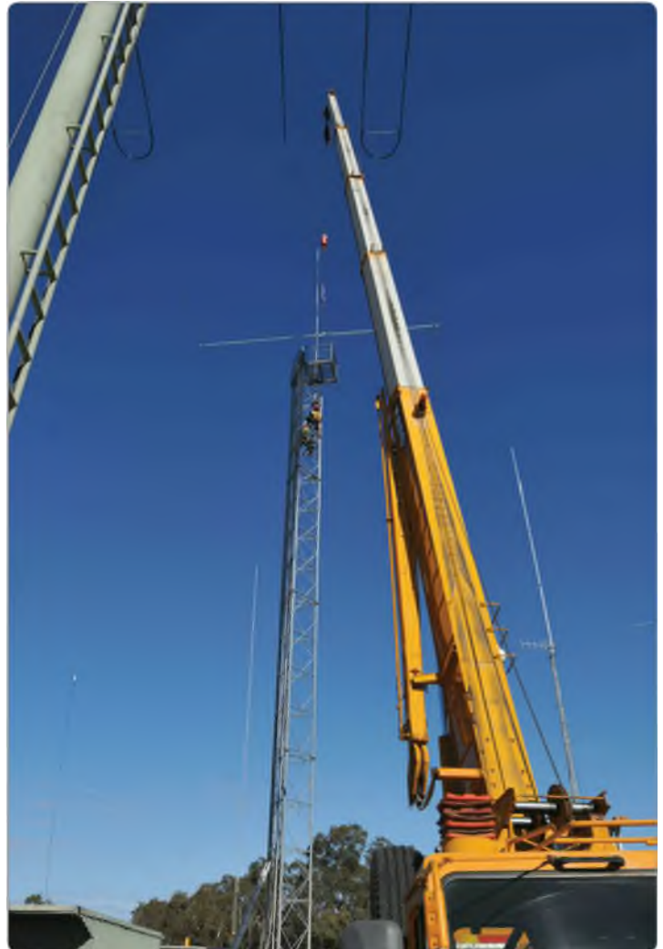
Photo 4: Crane needed for repair of 40 m beam.
