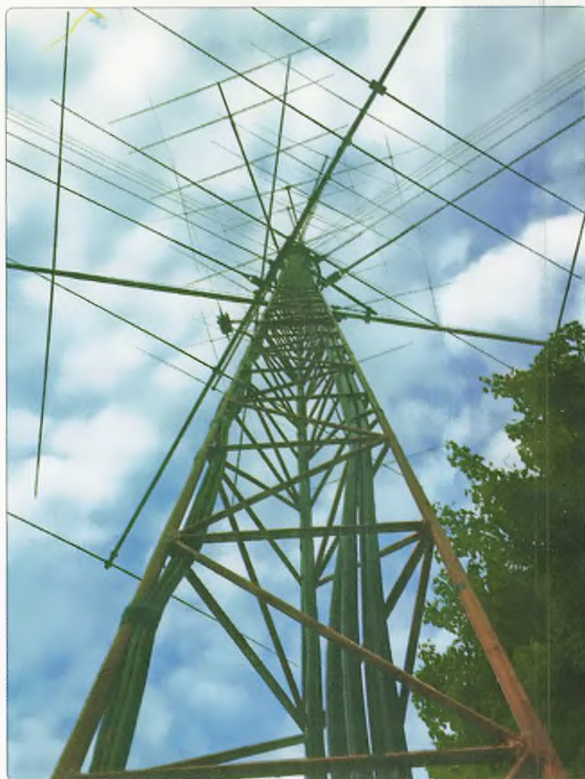
Photo 2: Looking up at one of the antenna arrays.
