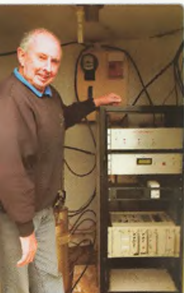
Photo 3: Col and Babies: A proud beacon constructor Col Hutchesson (VK5DK) stands by the new installation. From top: the beacons, the remote control receiver, the 146.8MHz repeater.
