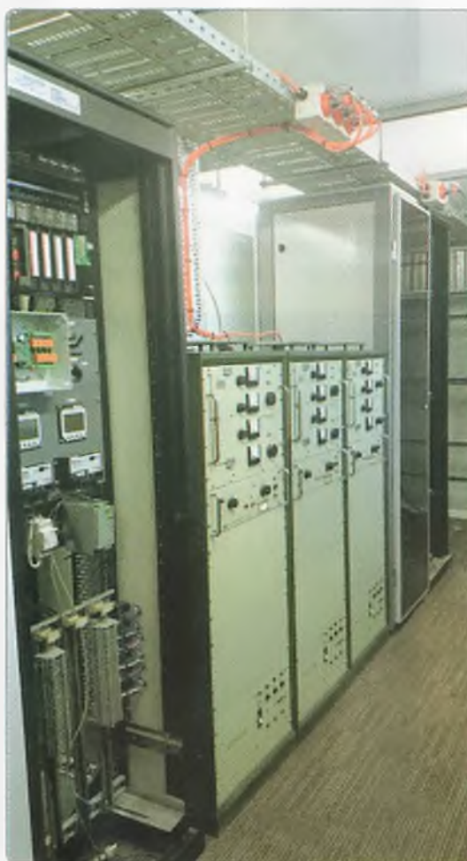
Photo 3: Control Room-work in progress.
