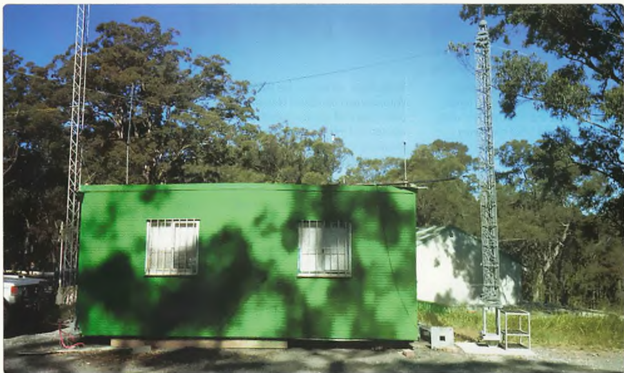
Photo 3: The new antenna is on the right of the building and compliments the original mast that supports the 70 cm repeater antenna.
