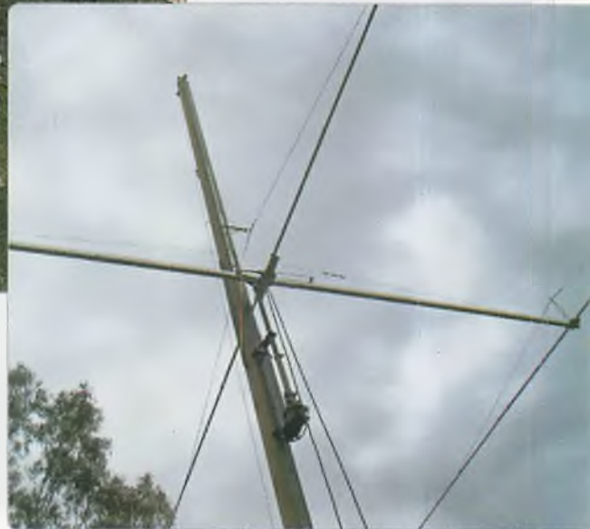
Photo 6: The stub mast assembling carrying a Yagi into position.
