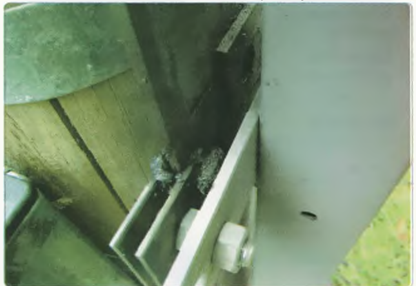
Photo 8: Detail of the carriage assembly on its guide track.
