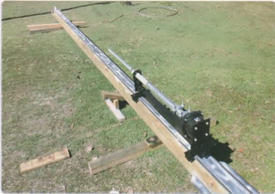
Photo 4: The rotator, stub mast and carriage in position on the mast prior to elevation.
