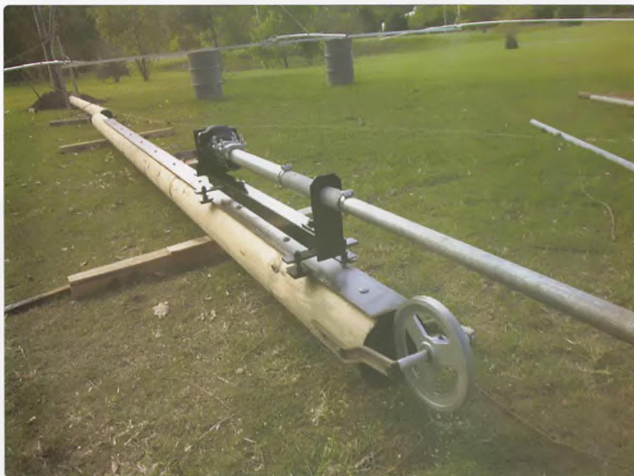
Photo 3: Another view of the stub mast and rotator carriage in position on the carrier rail.
