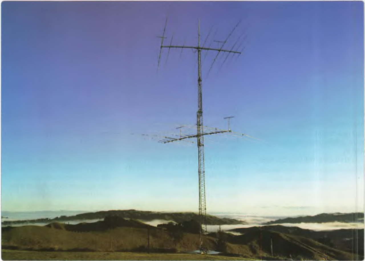
Photo 2: Multi band Yagi Stack, including 2 over 2 element on 40 m.
