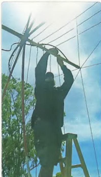
Photo 1: Travis disconnecting wires from centre post (Photo Lyn Battle VK4SWE).
