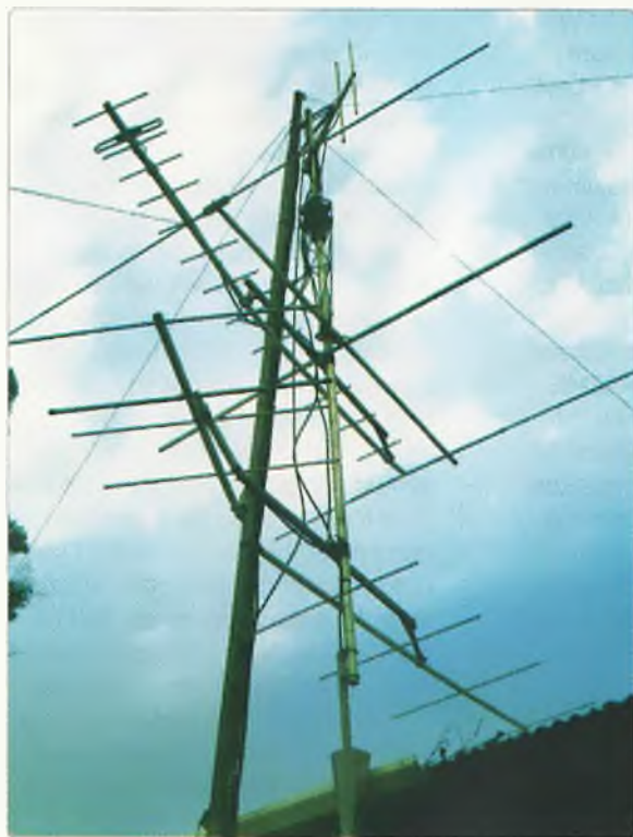
Photo 4: Significant Damage to Derek VK6DZ's Yagi antennas 25 May.
