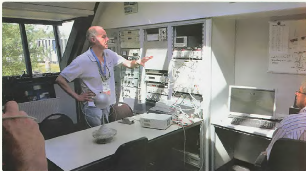
Photo 3: Jan PA3FXB demonstrating the PI9CAM EME installation.
