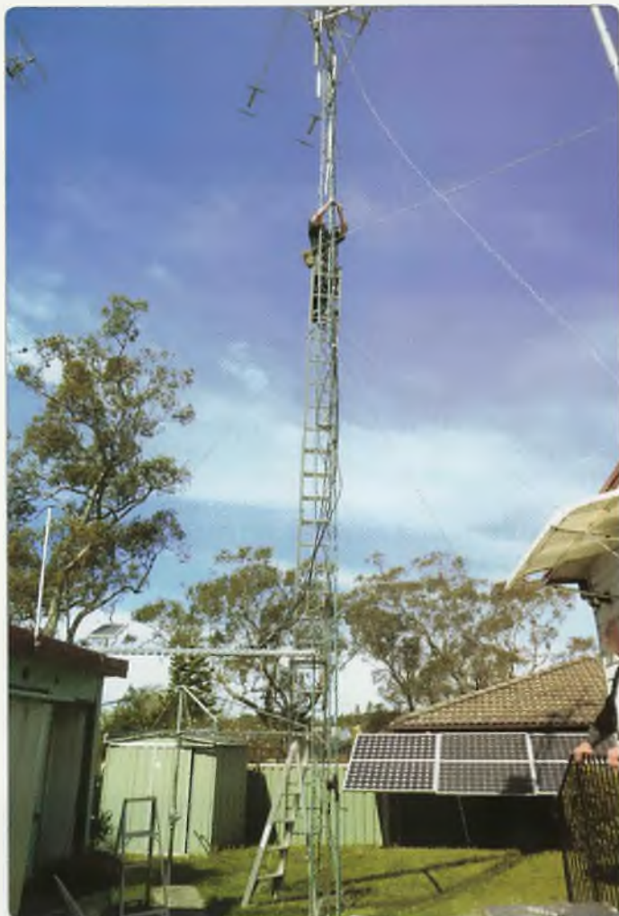
Photo 3: Installing the receiver and antenna on the tower.
