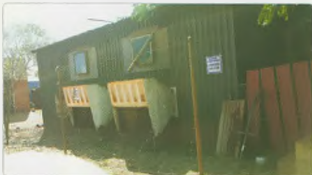
Photo 10: The rear of the transmitter hut at the De Grey site.
