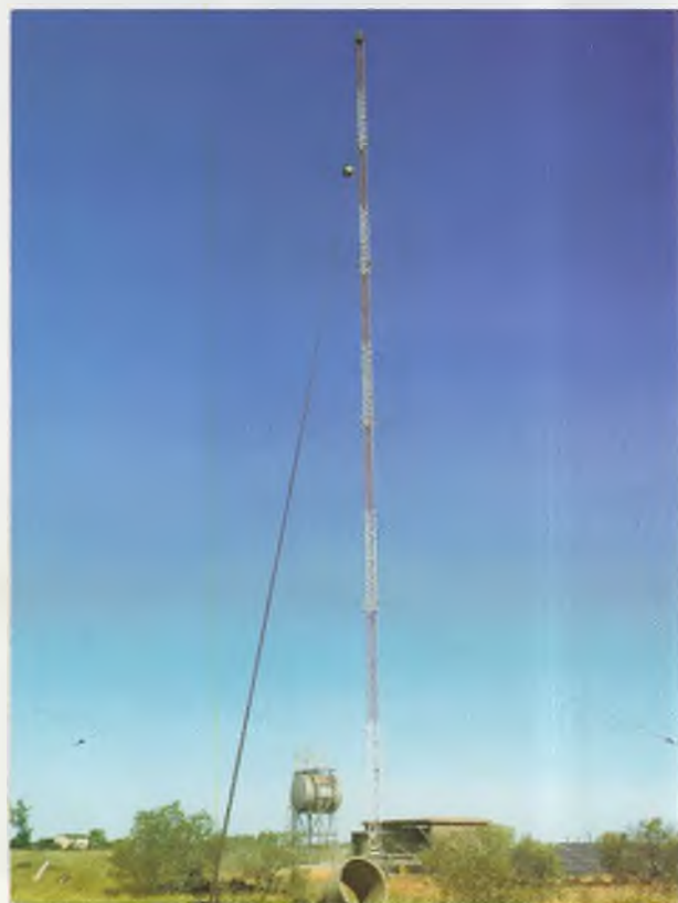
Photo 8: The antenna at the De Grey site.
