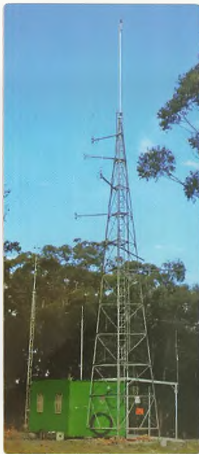
Photo 1: Overview of the Club mast.
