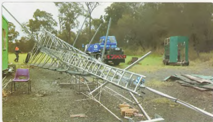
Photo 2: The mast whilst under construction.
