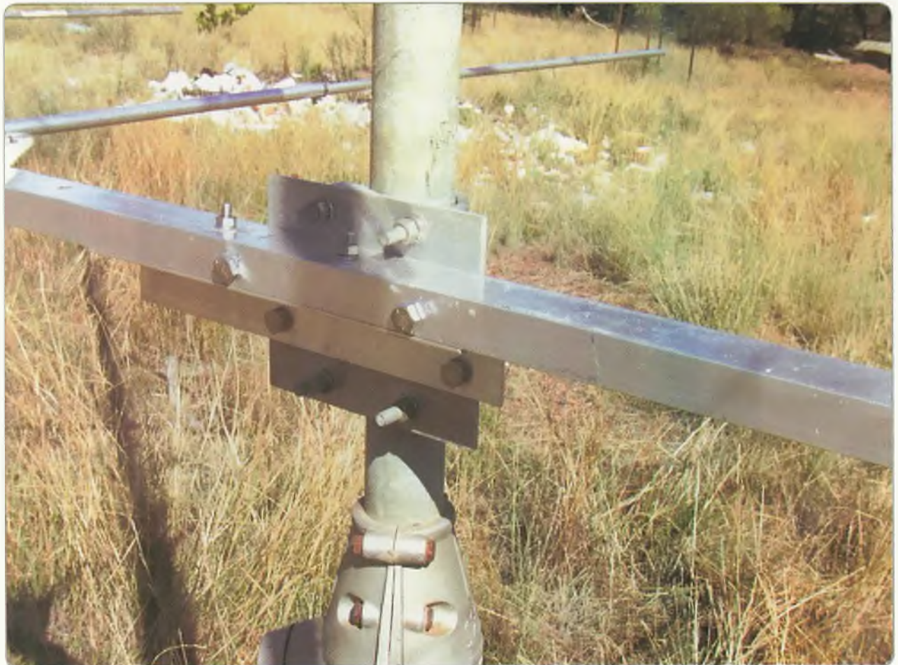
Photo 4: The mast to boom bracket.
