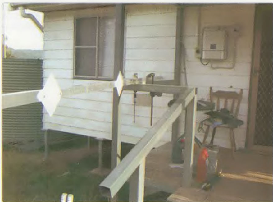
Photo 2: The boom with element mounting plates mounted.
