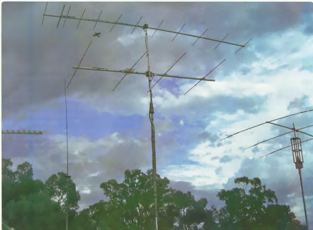
Photo 7: The Yagi mounted at my QTH.
