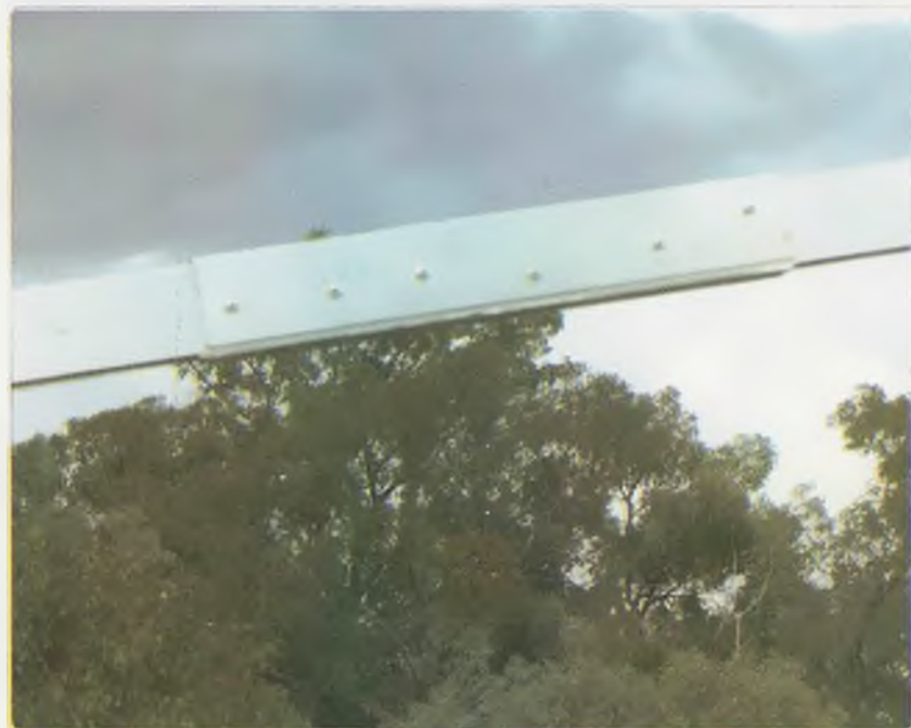
Photo 1: Detail showing the join in the boom.
