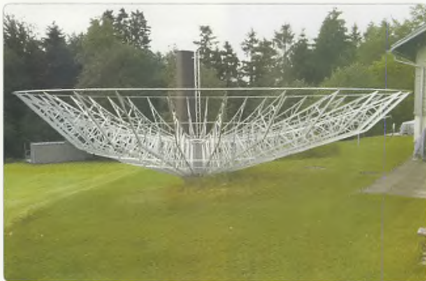
Photo 4: Erich OE9ERC's new 12 metre Dish under construction.
