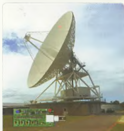
This month's cover: Main picture is a 6 GHz 27 metre diameter dish used for Moonbounce EME communications attempt.. See VK6 News on page 49 for details.
