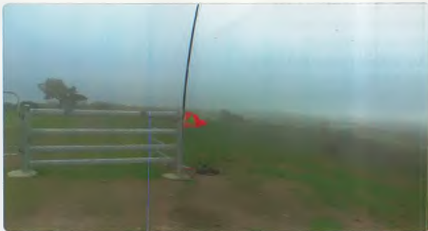
Photo 3: The antenna support lashed to the fence post.
