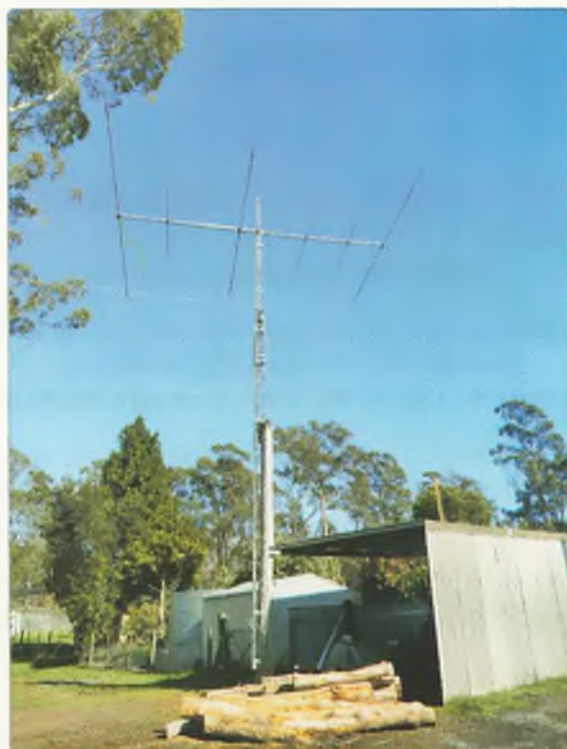
Photo 2: The erected aerial.
