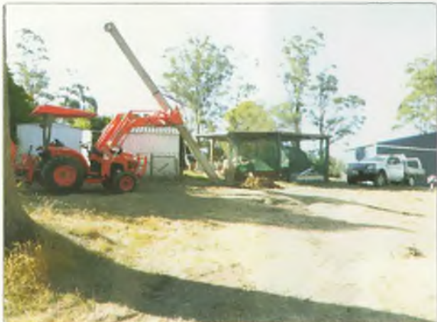
Photo 1: Raising the aerial with the tractor and pole.
